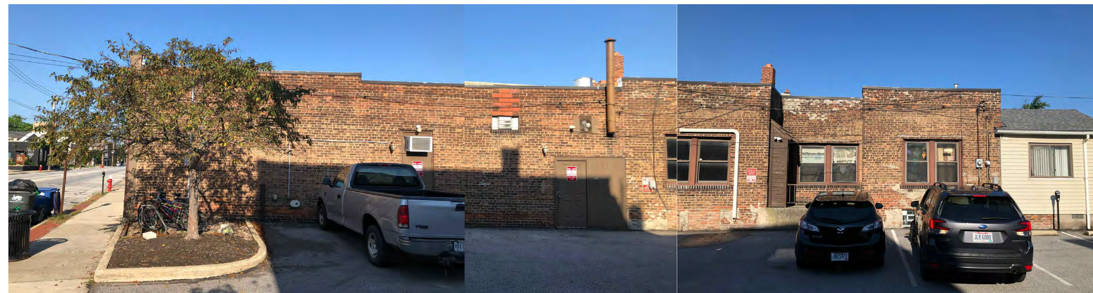
6 A2-00 EXISTING CONDITIONS SIDE (EAST) CORNER AT CITY PARKING LOT SCALE: N.T.S.
