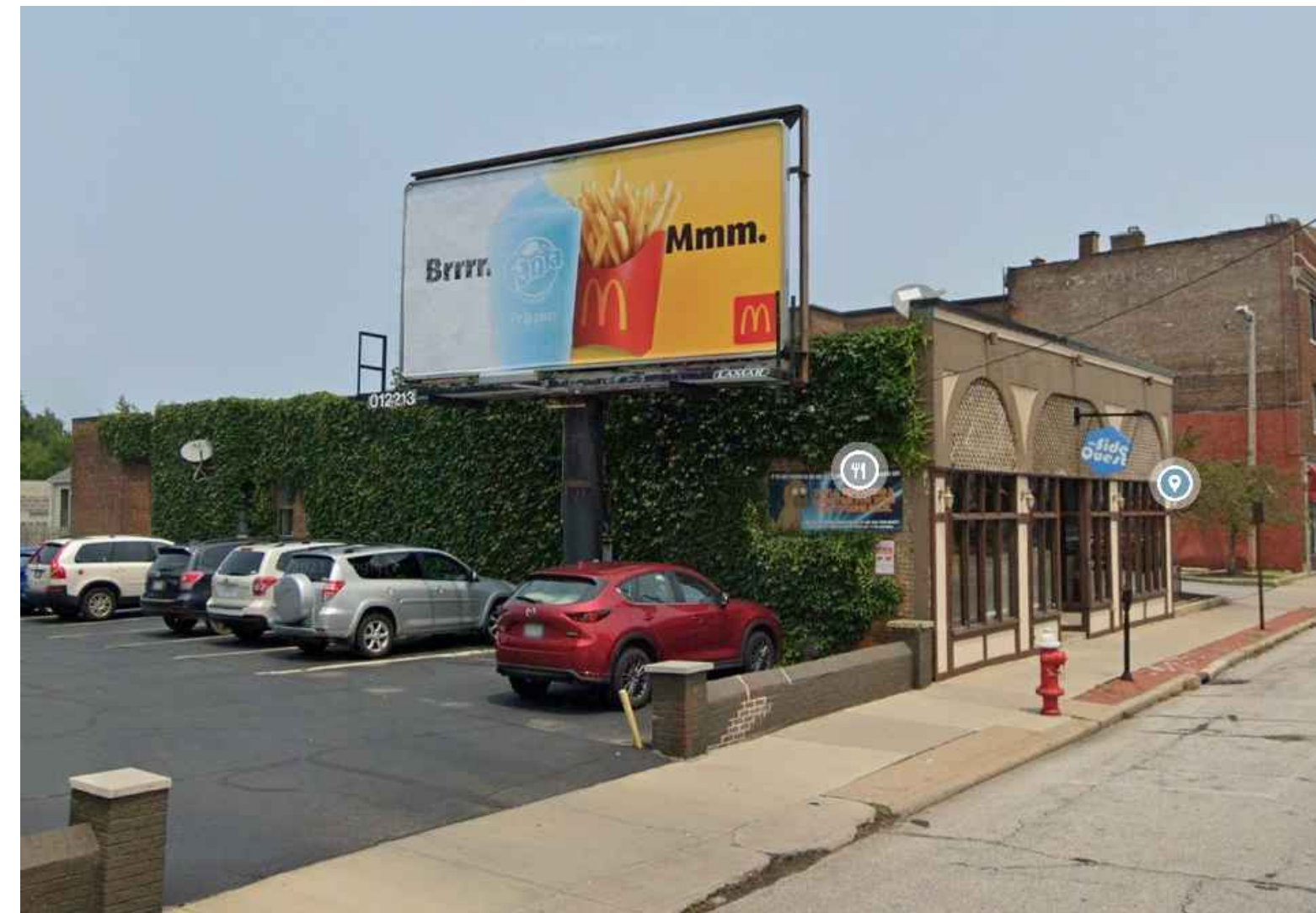
2 A2-00 EXISTING CONDITIONS FRONT (SOUTHWEST) CORNER AT DETROIT SCALE: N.T.S.
