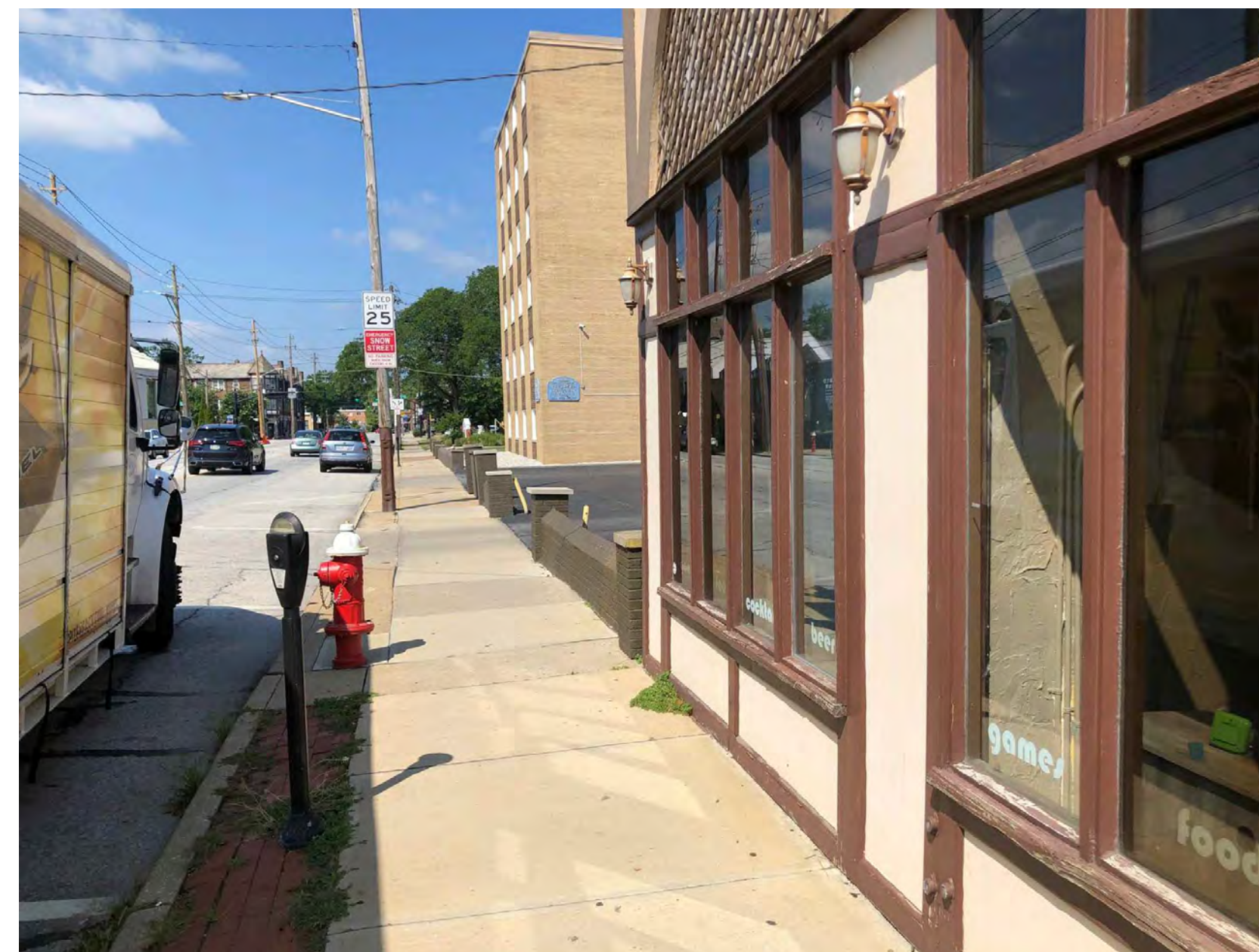
4 A2-00 EXISTING CONDITIONS FRONT (SOUTH) ELEVATION AT SIDEWALK DETAIL SCALE: N.T.S.
