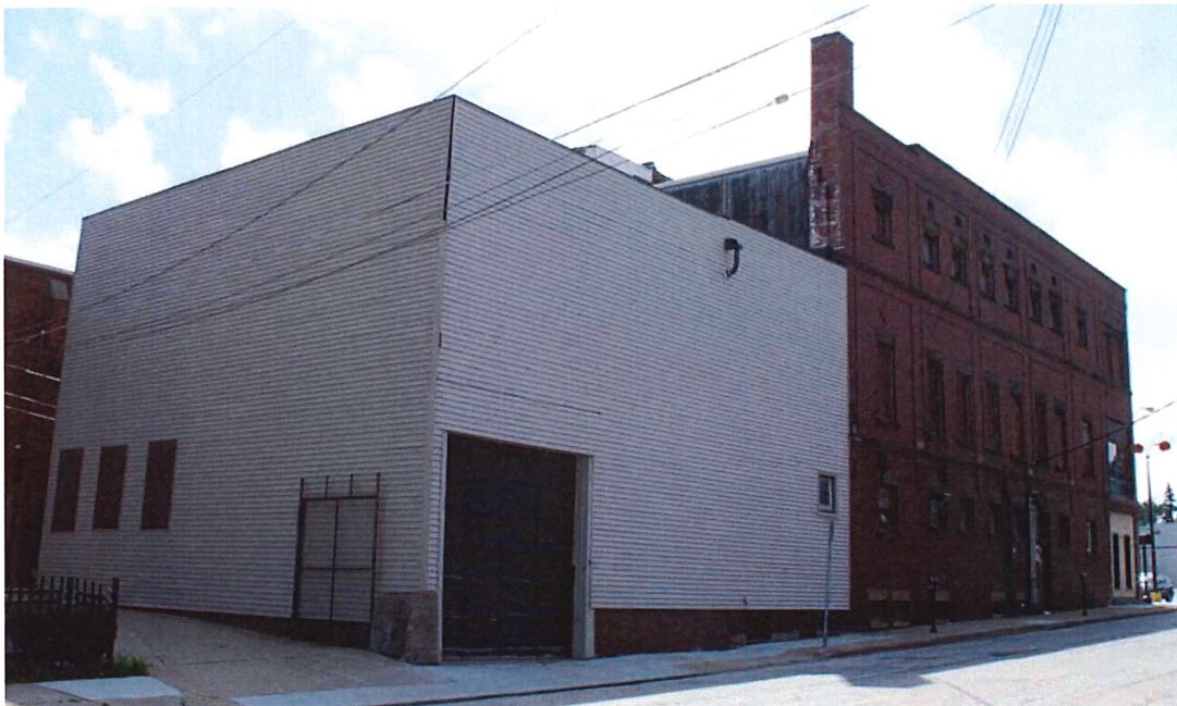
Photo 3: North and West Elevations, 2017.
