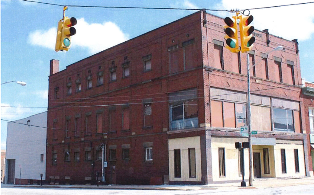
Photo 2: South and West Elevations, 2017.
