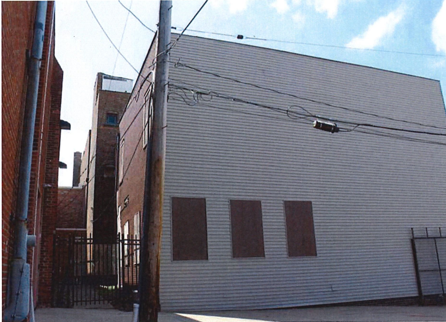
Photo 4: North and East Elevations, 2017.
