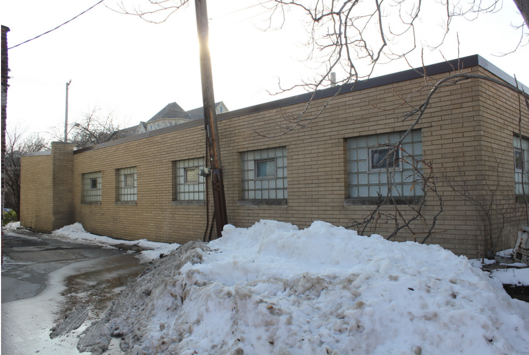
Photo 10: East elevation, looking southwest, 2018.
