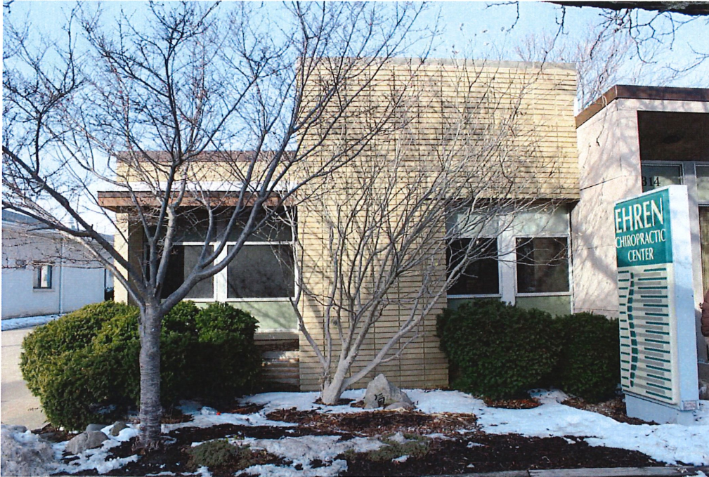
Photo 6: South elevation, detail of western section, looking north, 2018.
