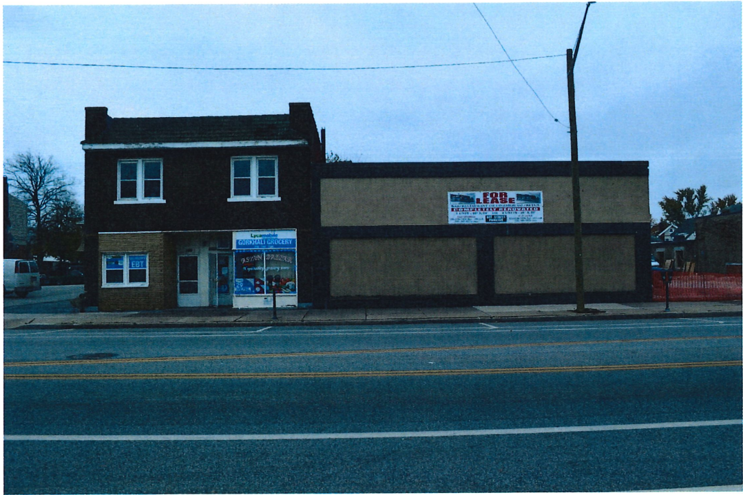
Front View of Building at 13415 Madison Avenue, Lakewood
