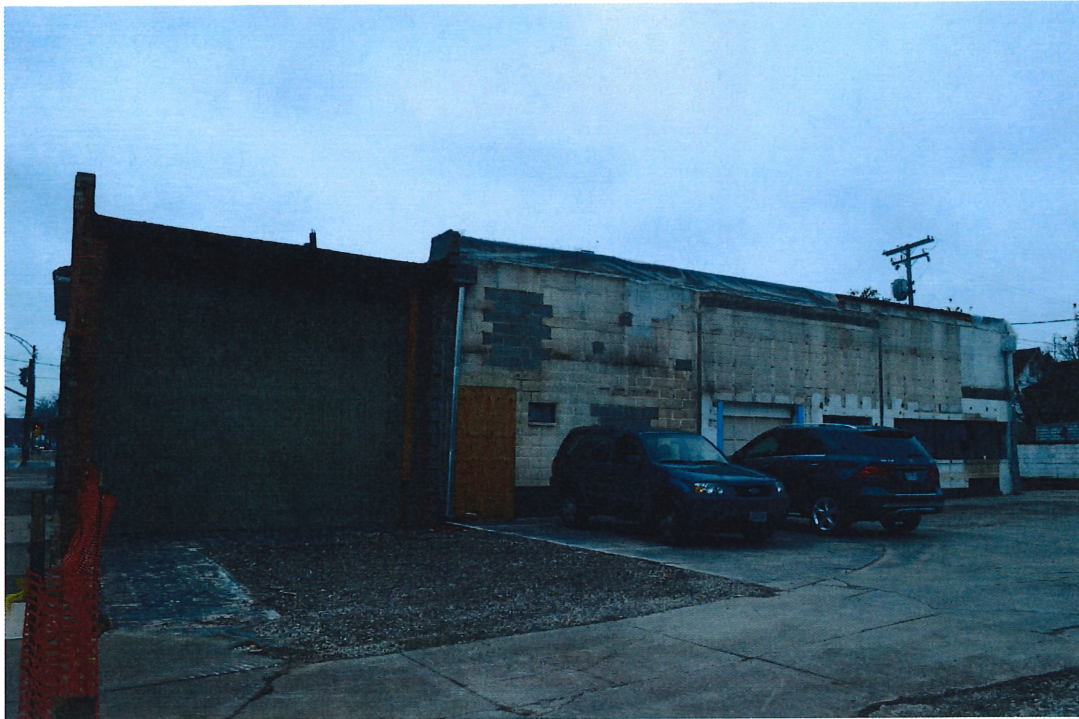
Side View of Building at 13415 Madison Avenue, Lakewood
