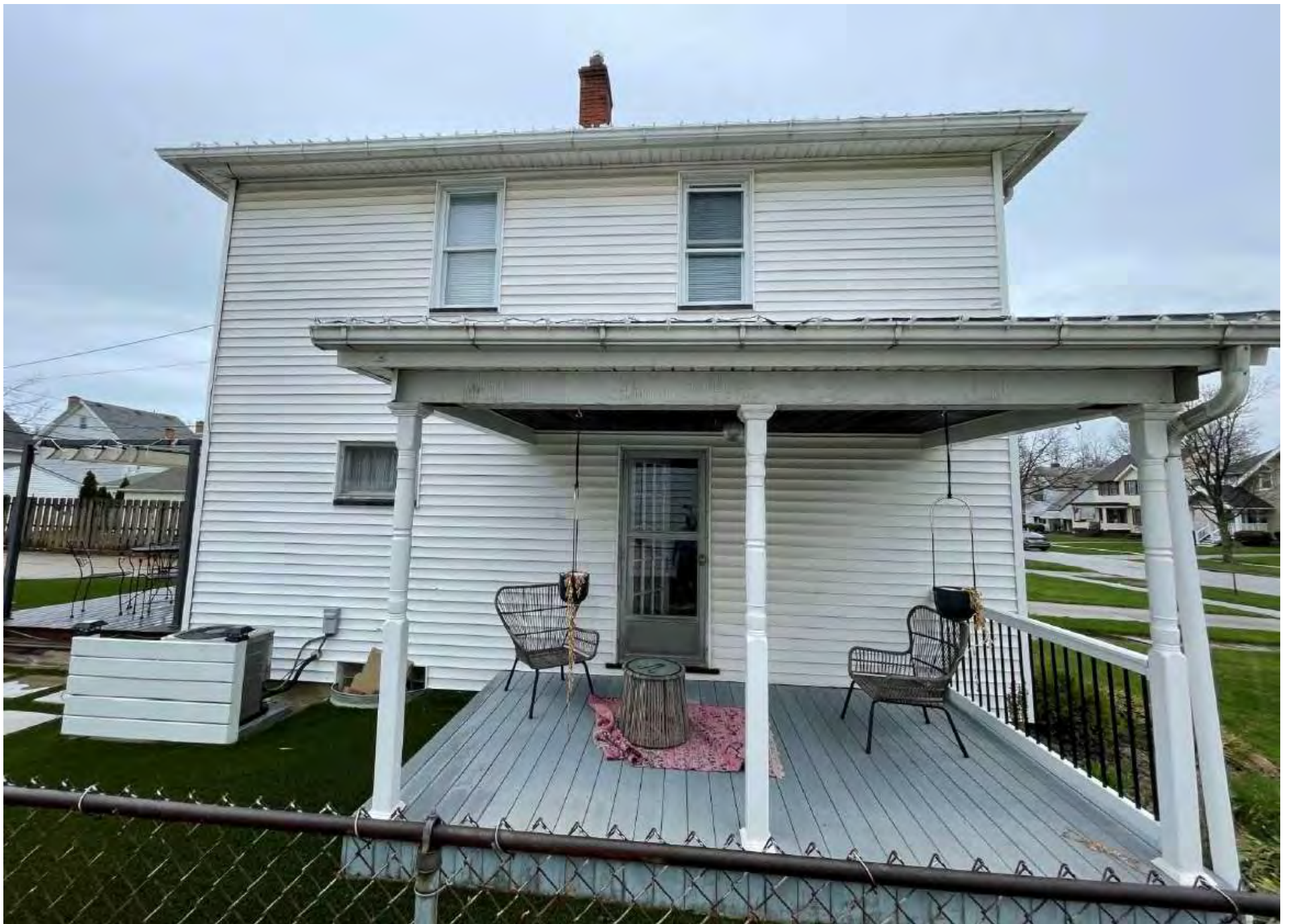
Docket No. 06-29-22 (2064 Lincoln) Renovation of Side Porch
