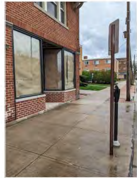
Existing Photo Looking West
