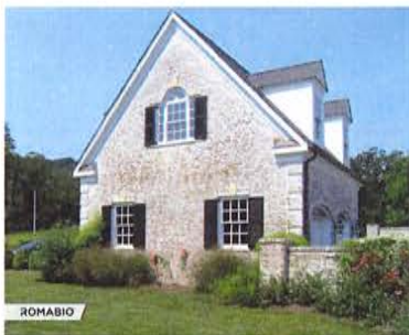
LIME WASHED BRICK WITH WHAT APPEARS TO BE STUCCO DORMERS AND AGING COPPER GUTTERS AND DOWNSPOUTS
