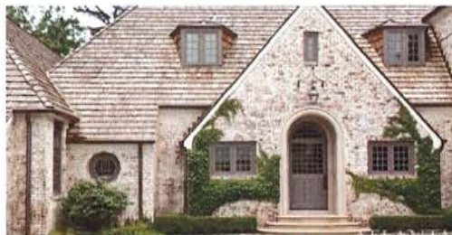
LIME WASHED BRICK WITH SHAKE SHINGLE ROOF AND WHAT APPEARS TO BE AGING COPPER GUTTER AND DOWNSPOUTS
