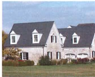
LIME WASHED BRICK WITH WHAT APPEARS TO BE STUCCO DORMERS
