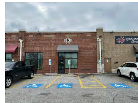
IMPOSED DRAWINGS ARE NOT TO EXACT SCALE AND ARE PROVIDED FOR REPRESENTATIONAL PURPOSES ONLY.
