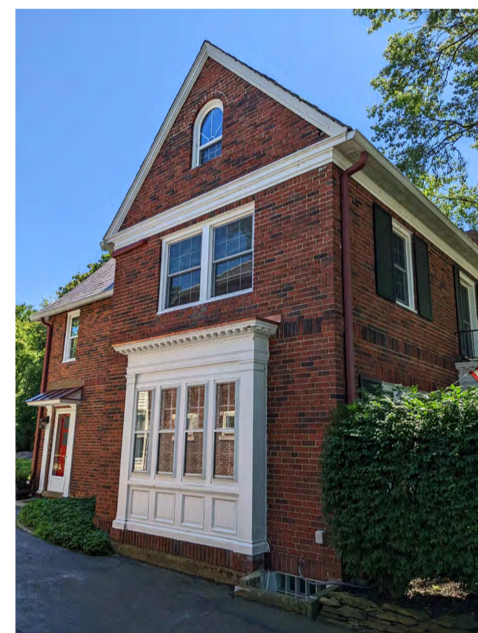
Detailing Reference Photo (North Side of Home)
