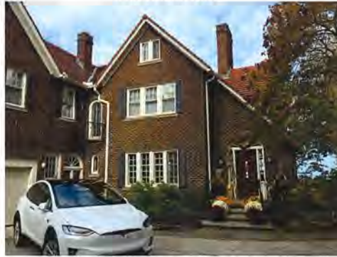
NEW PROPOSED ENCLOSED FRONT ENTRY PORCH. REPLACE EXISTING FRONT DOOR WITH WINDOWS TO MATCH THE EXISTING SIDES AND REAR PARLOR WINDOWS.
