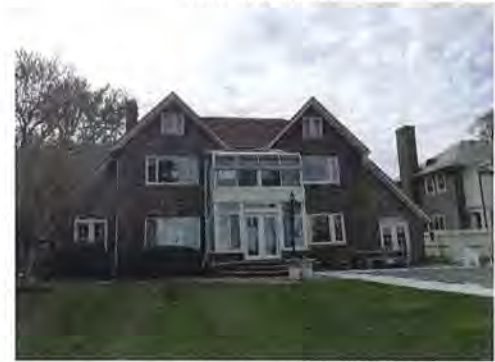
REMOVE EXISTING GLASS SOLARIUM AND REPLACE WITH NEW GREAT ROOM / DINING ROOM ADDITION WITH REAR COVERED TERRACE.
