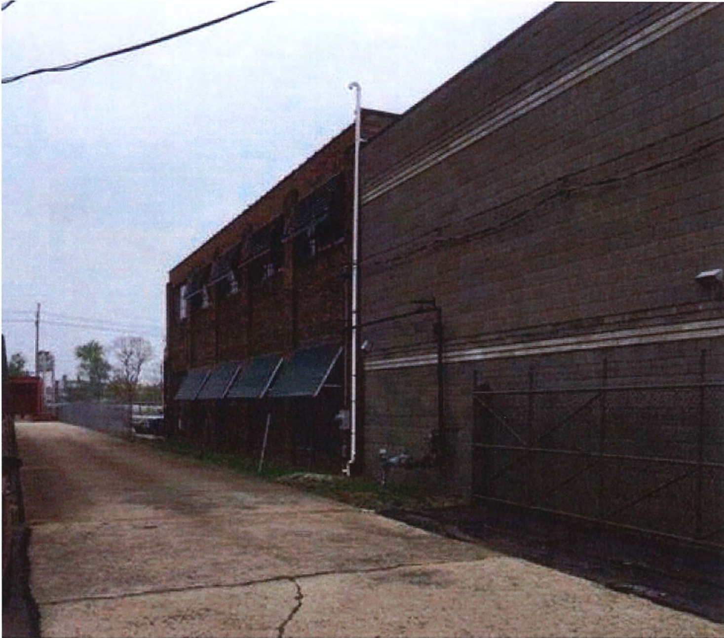
Buildings to Be Demolished
