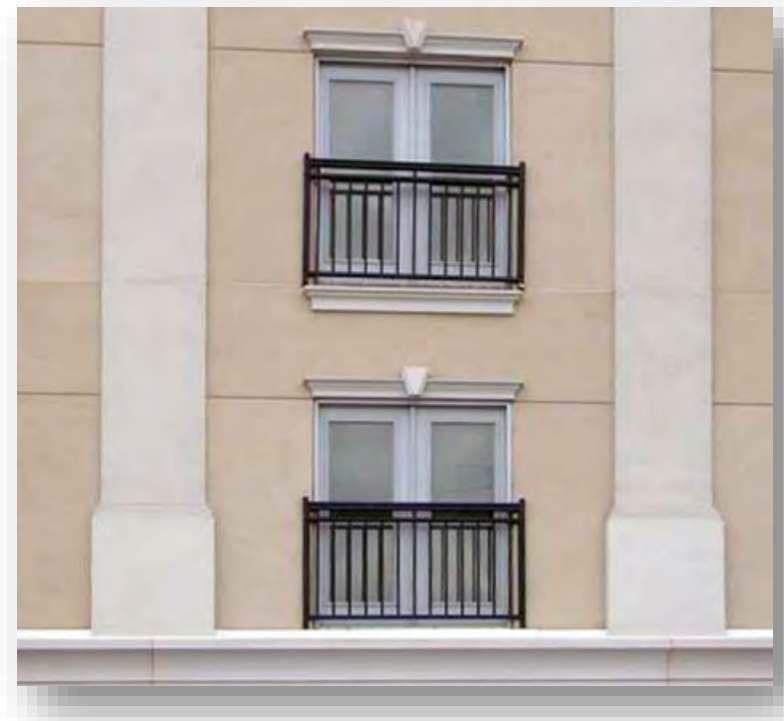
ALUMINUM RAILING AT BUILDING BALCONIES
