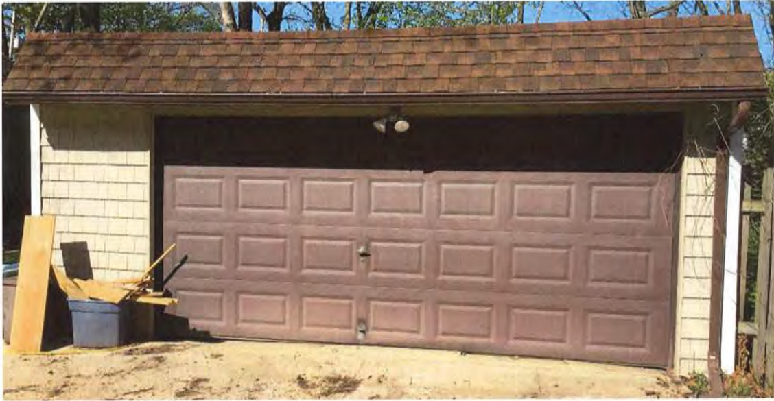
Current two car garage that would be torn down.
