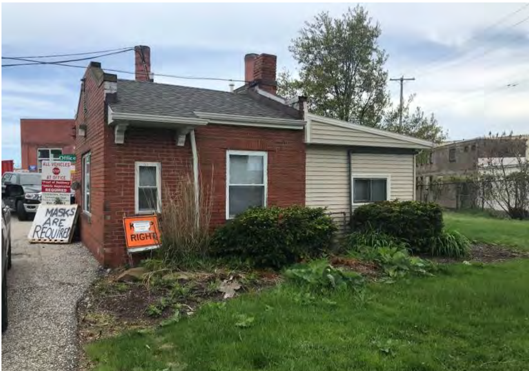
Picture 4: Existing recycling check-in building (to be removed)
