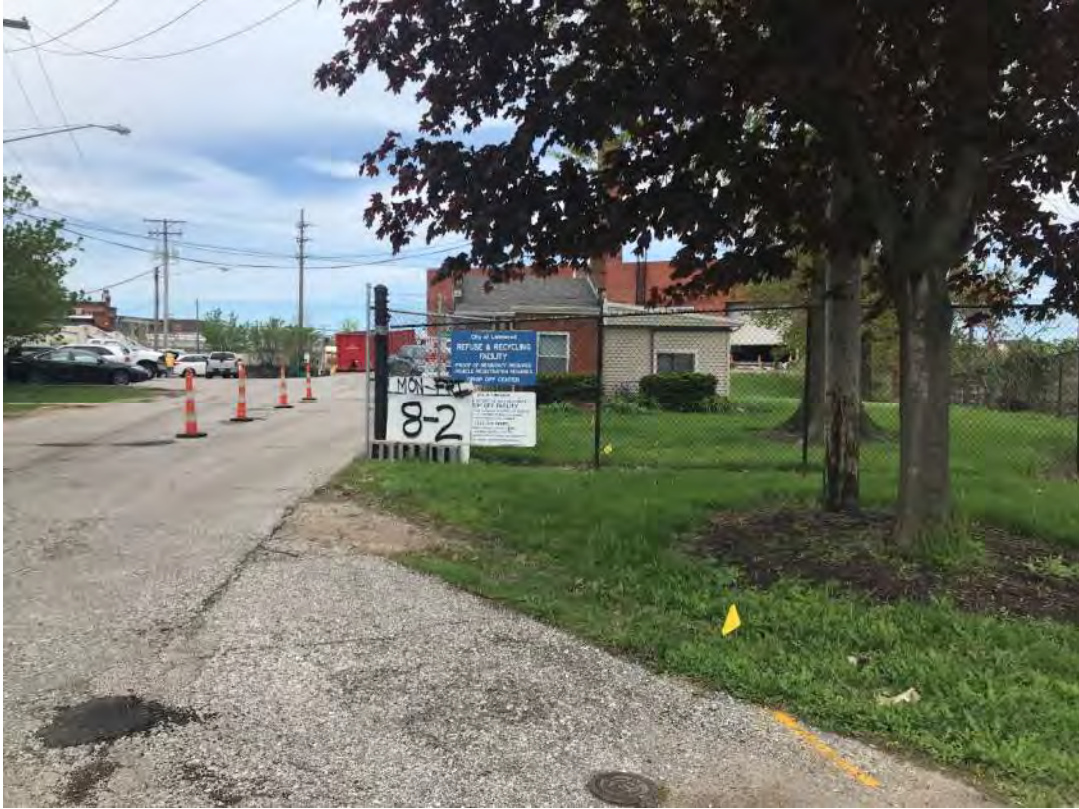
Picture 3: Existing recycling check-in building (to be removed) looking north
