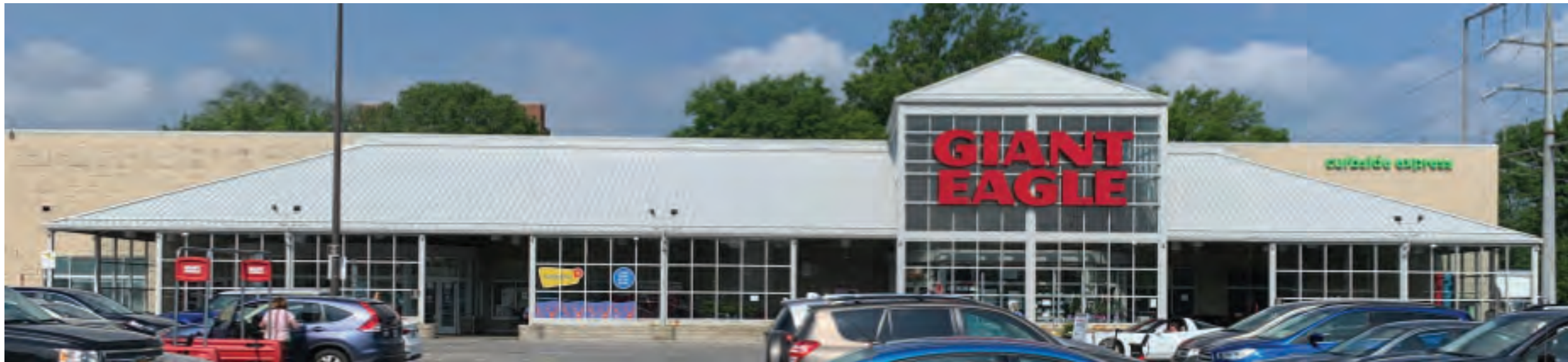
EXISTING SIGNAGE: GIANT EAGLE DIMENSIONS - 8'-6" H x 23'-4" W EXISTING SIGN SQ FT: 198.3
