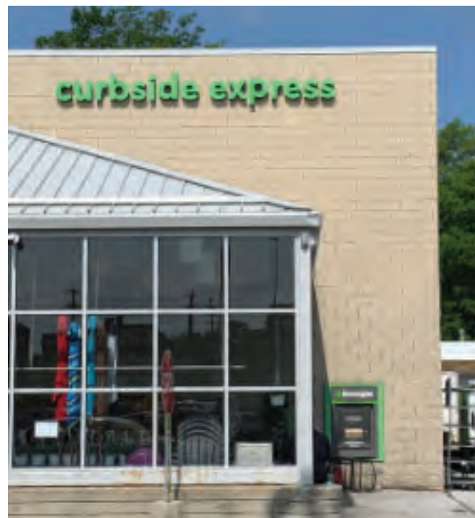
EXISTING SIGNAGE DIMENSIONS - 1'-1 1/2" H x 17'-2 1/2" W EXISTING SIGN SQ FT: 19.4
