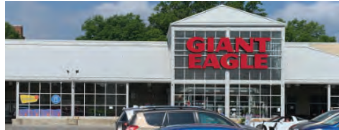
EXISTING SIGNAGE DIMENSIONS - 8'-6" H x 23'-4" W EXISTING SIGN SQ FT: 198.3
