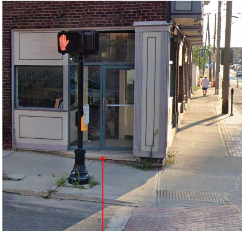
SPACE 1 ENTRY: 5.5" - 10" STEP FLOOR ELEVATION 679.3
