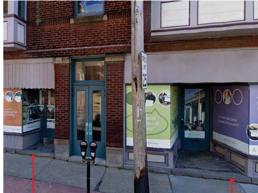
SPACE 2 ENTRY: +/-5" STEP FLOOR ELEVATION 678.9 (-4 1/2")
