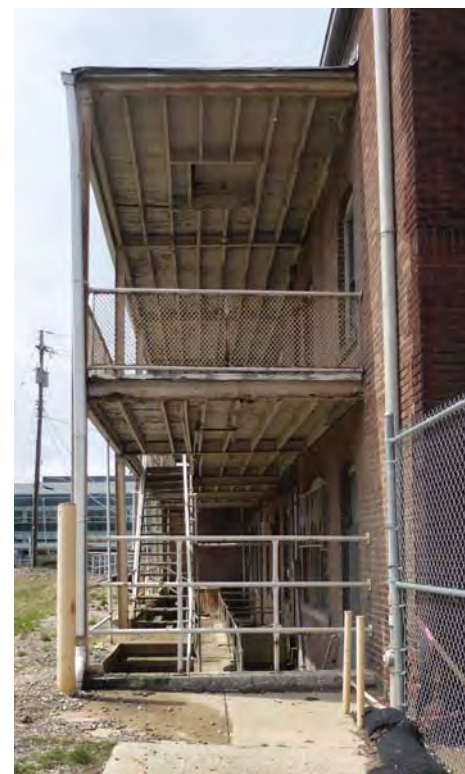
South facade walkway
