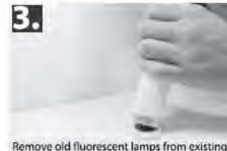
3. Remove old fluorescent lamps from existing lamp sockets.
