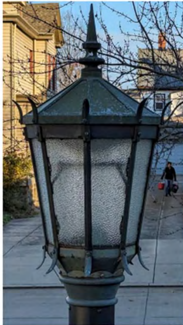
EXISTING LIGHT FIXTURE
