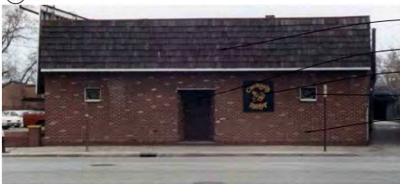
2 HISTORIC FACADE - REMODELED BRICK LATE 1970S - CUCKOO'S NEST SCALE: N.T.S.
