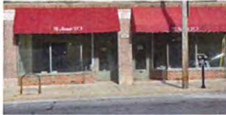
EXISTING STREET VIEW
