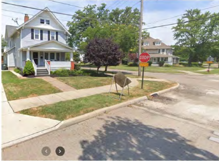
1346 MATHEWS AVE LAKEWOOD, OH. 44107
