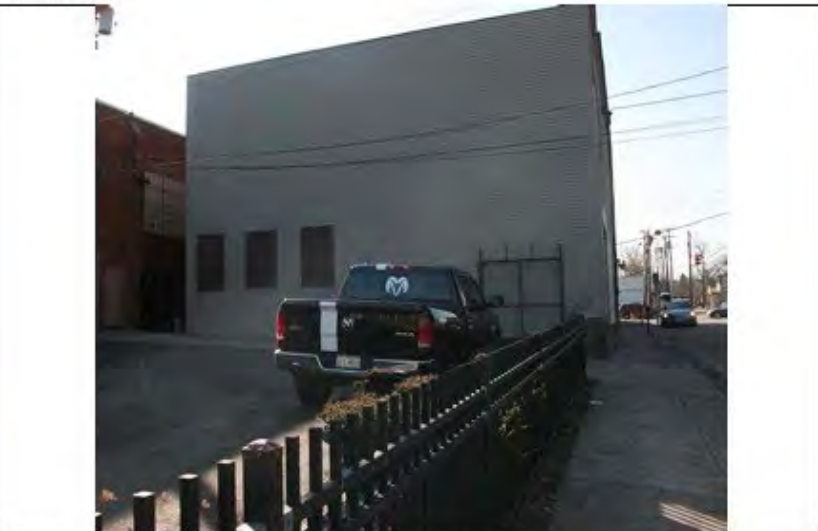
Photograph 4 – View of rear of property, looking south.
