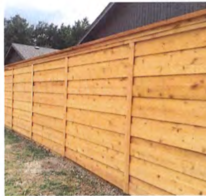
6' horizontal board on board wood fence
