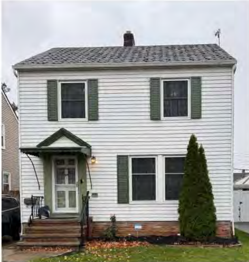
EXISTING FRONT FACADE
