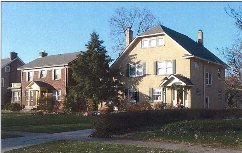
Neighboring Home Design – Erie Cliff Drive
