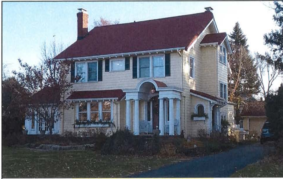
Neighboring Home Design – Erie Cliff Drive
