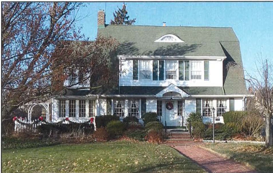
Neighboring Home Design – Erie Cliff Drive
