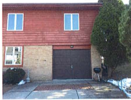
TWO STORY PORTION OF HOUSE INDIANOLA AVE.
