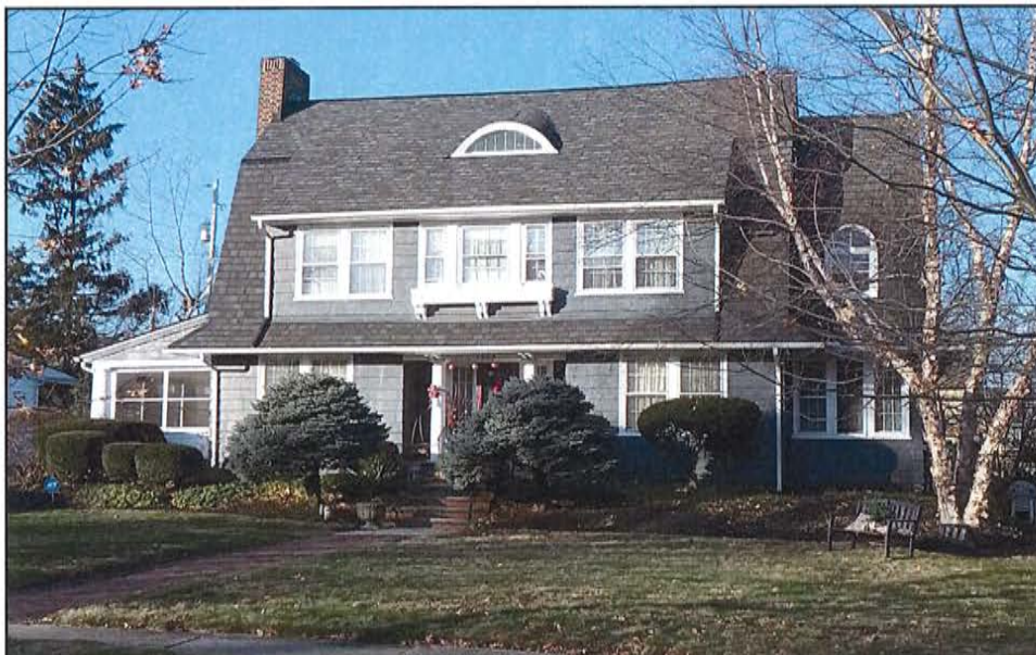
Neighboring Home Design – Erie Cliff Drive
