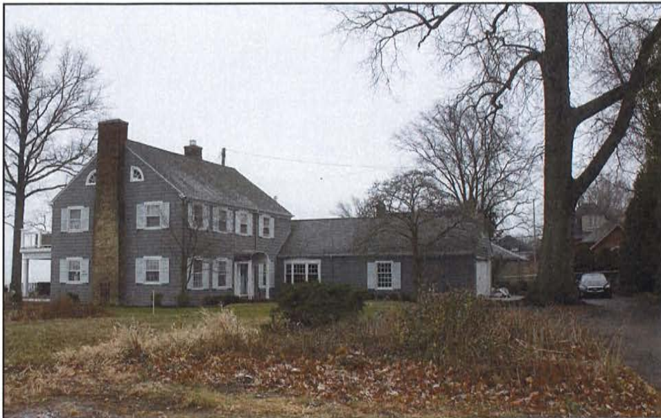
Neighboring Home Design – Erie Cliff Drive
