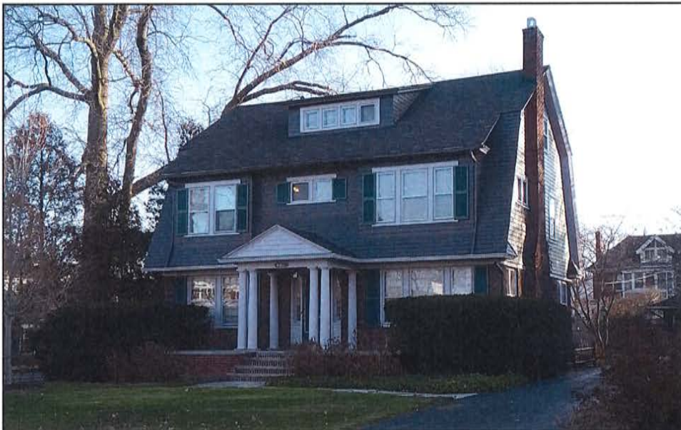
Neighboring Home Design – Erie Cliff Drive
