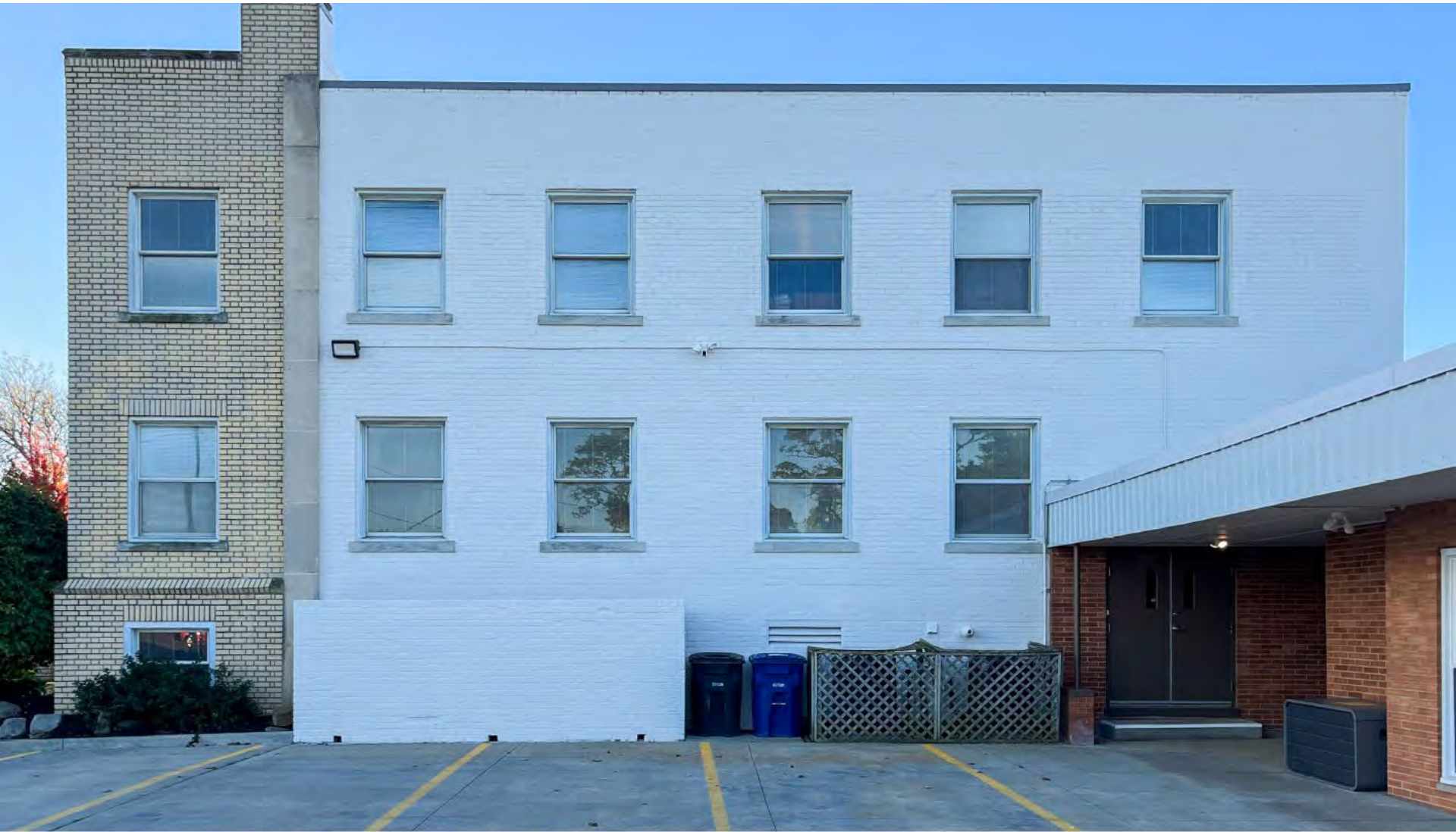
NORTH ELEVATION OF SANCTUARY BUILDING & EAST ELEVATION OF ANNEX ADDITION
