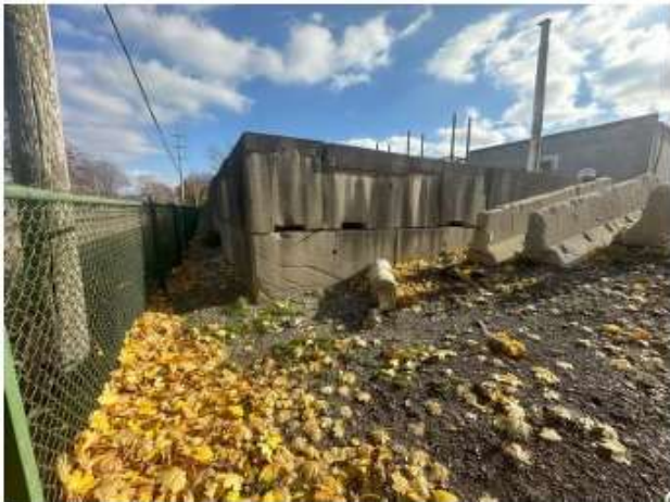
JERSEY BLOCK WALL - NORTHWEST CORNER
