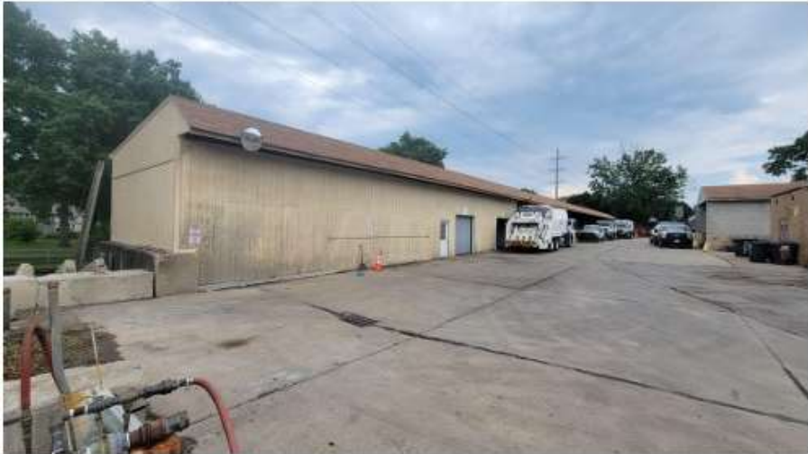
FORMER STORAGE BUILDING
