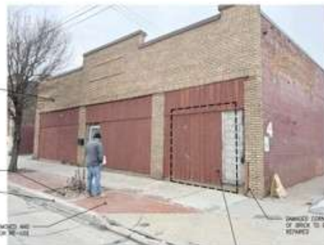
C EXISTING EAST ELEVATION A101 NO SCALE
