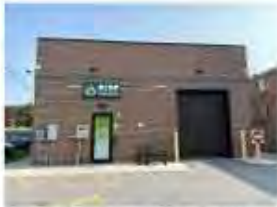
EXISTING EXTERIOR PHOTO FROM THE NORTH
