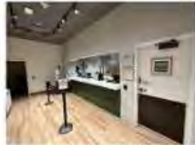
EXISTING INTERIOR PHOTO OF RETAIL AREA
