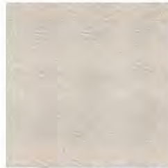
Existing EIFS Cladding
