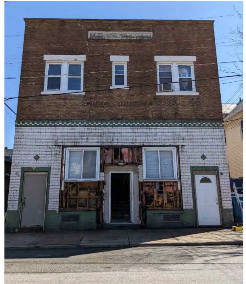
Existing Brick Found
