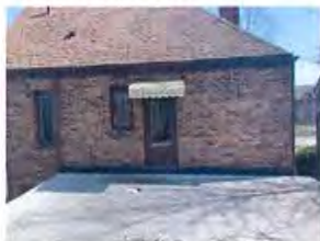
View from garage roof:
