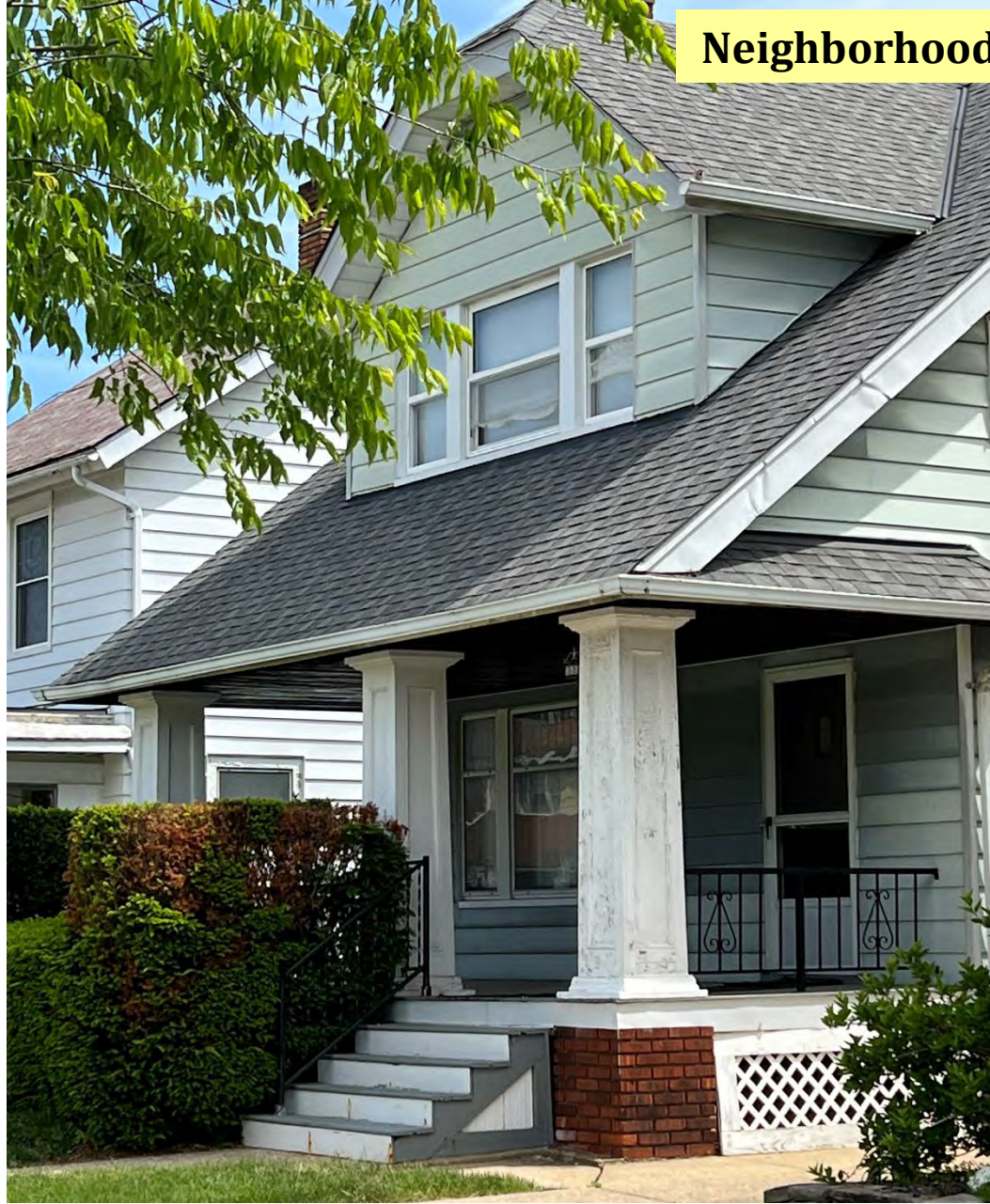
Docket No. 06-49-23 (2083 Wyandotte) Front Porch Reconstruction/Renovation
