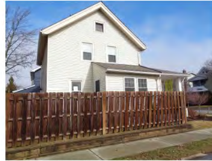
EXISTING SOUTH SIDE OF HOUSE HTS:
