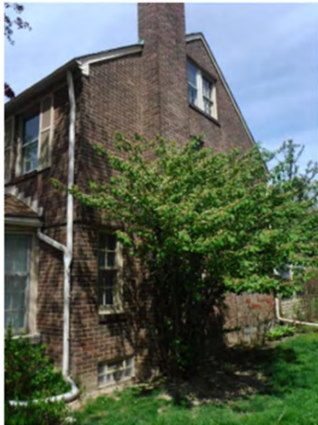
EXISTING PHOTO VIEWING NORTHWEST
