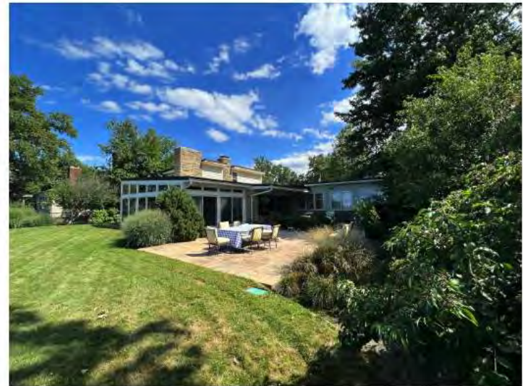
Existing structure, backyard view, showing mature vegetation
