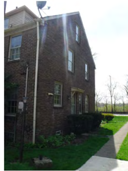
EXISTING PHOTO VIEWING SOUTHEAST
