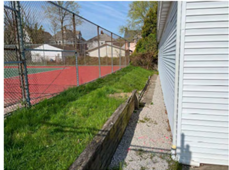
Looking west in between the storage building and northern-most tennis court
