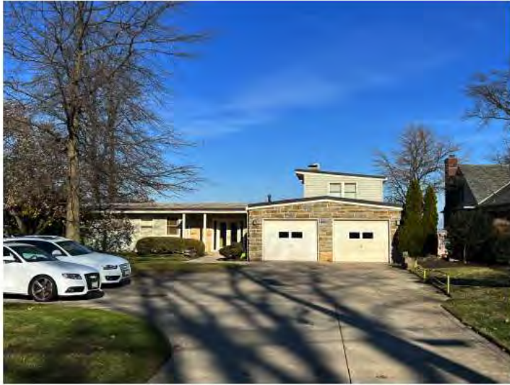
Existing structure, as seen from Edgewater Drive
