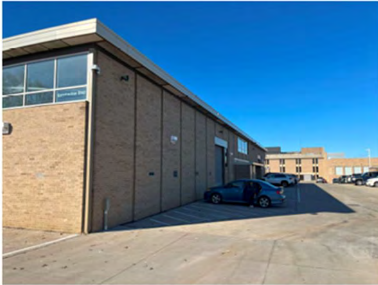
Looking north along the east elevation of the D Building
