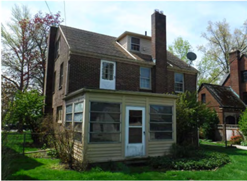
EXISTING PHOTO VIEWING SOUTHWEST
