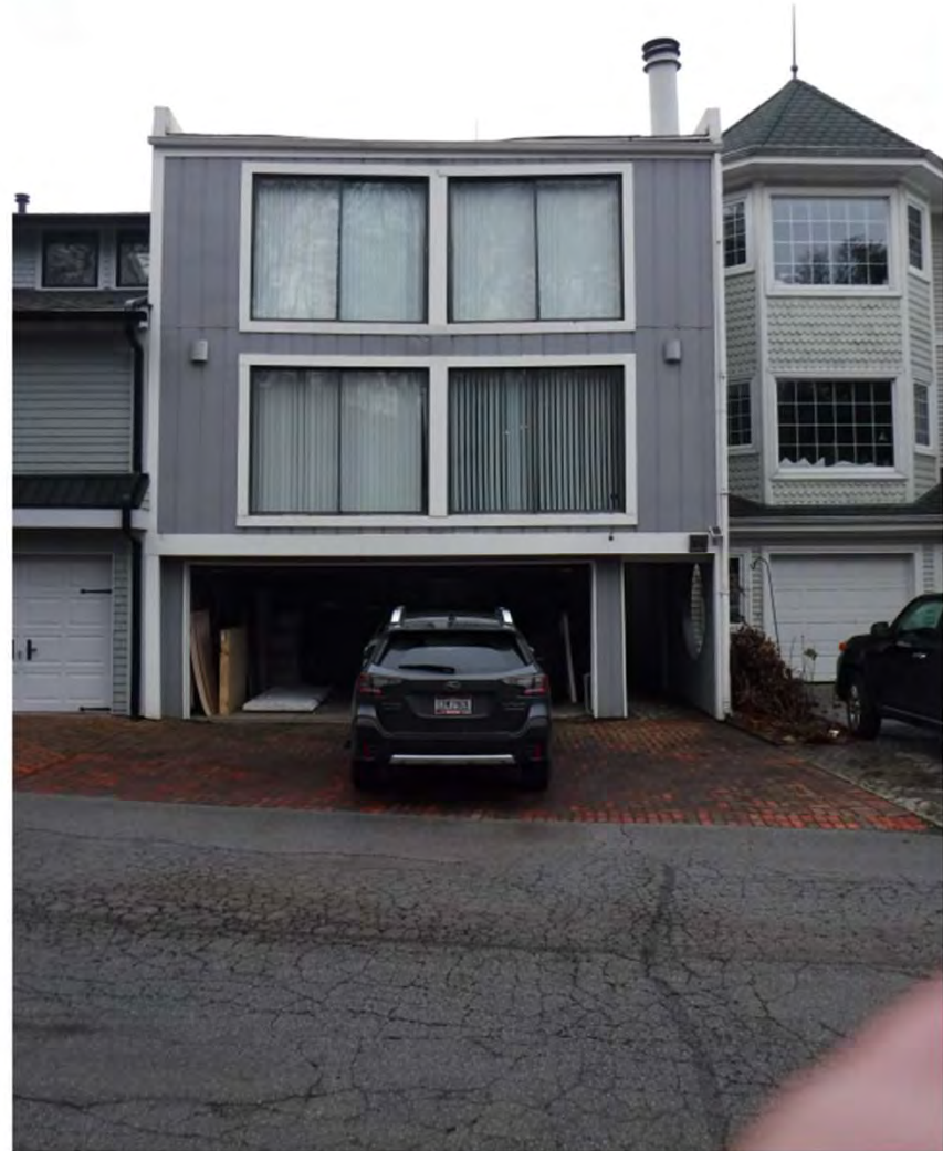
EXISTING CONDITIONS PHOTO VIEWING WEST N.T.S.
