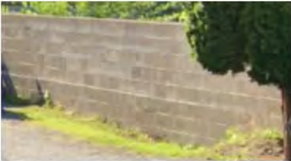
Existing 7'-0" Masonry Wall
