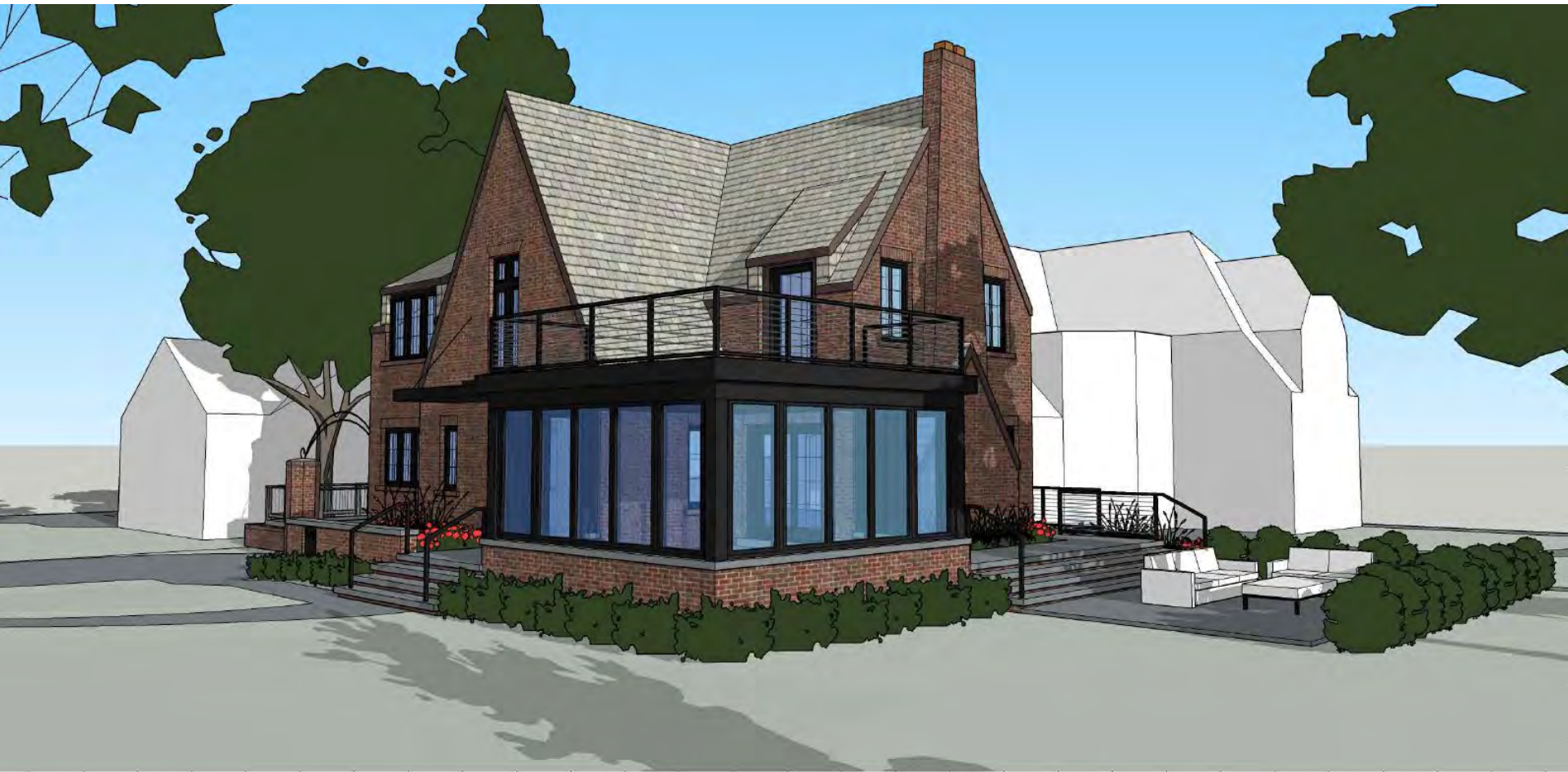
View from Corner of Cliff Drive & Wilbert Avenue
