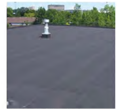
TORCH DOWN ROOFING
