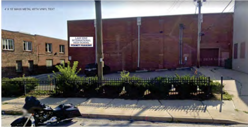
Parking around the corner. The Sign will be mounted with "Tapcon" screws into the brick mortar . Screw heads will be covered with print material.
