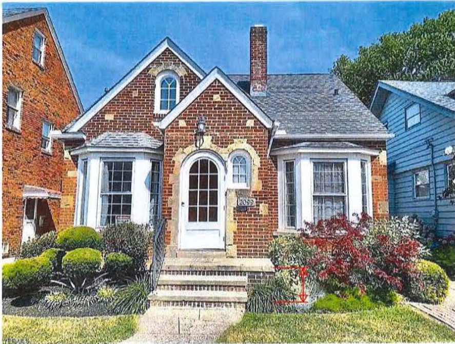
2099 OLIVE AVE. EXISTING HOUSE STRUCTURE
