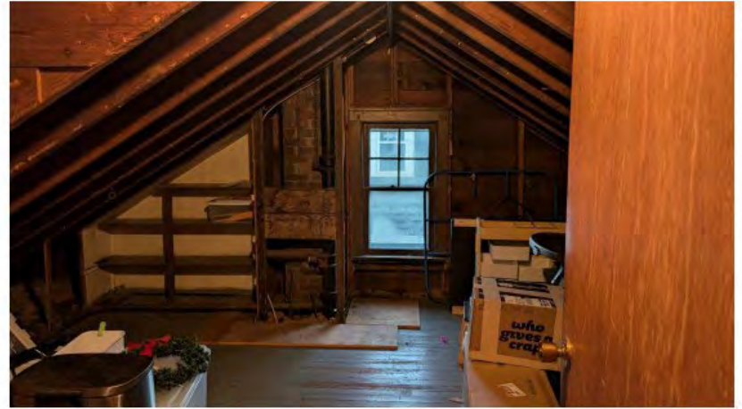
Existing unfinished attic space
