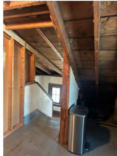
Existing stairs to attic
