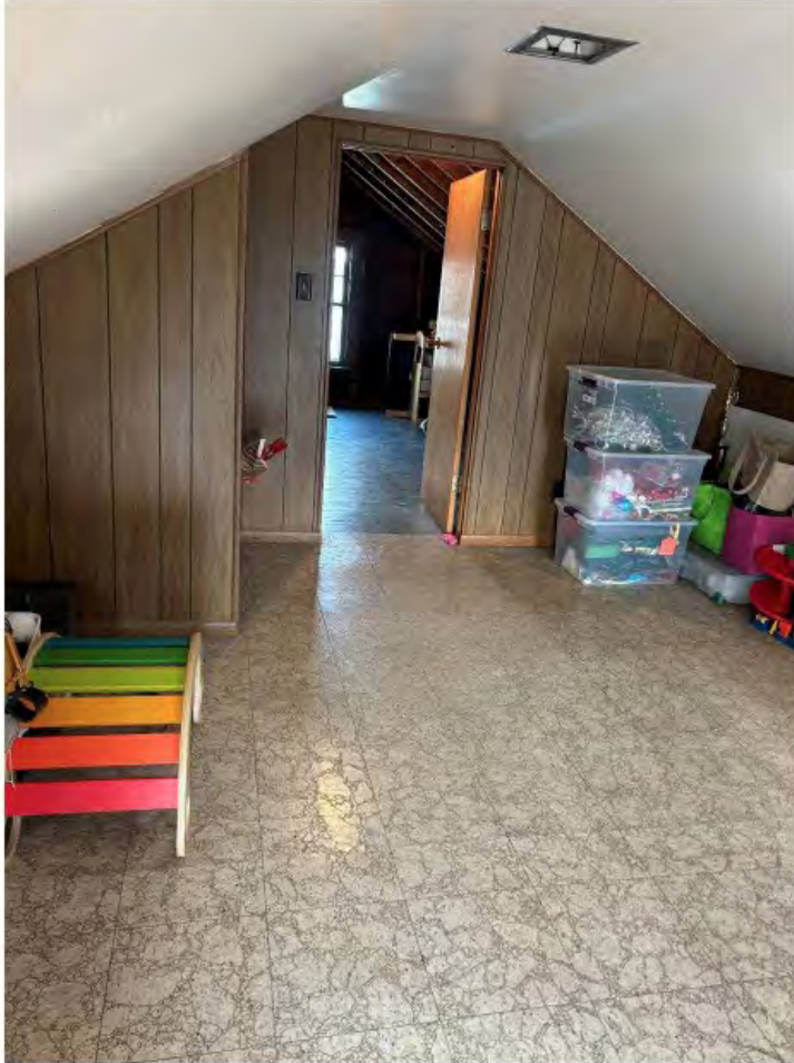
Existing finished attic space 1
