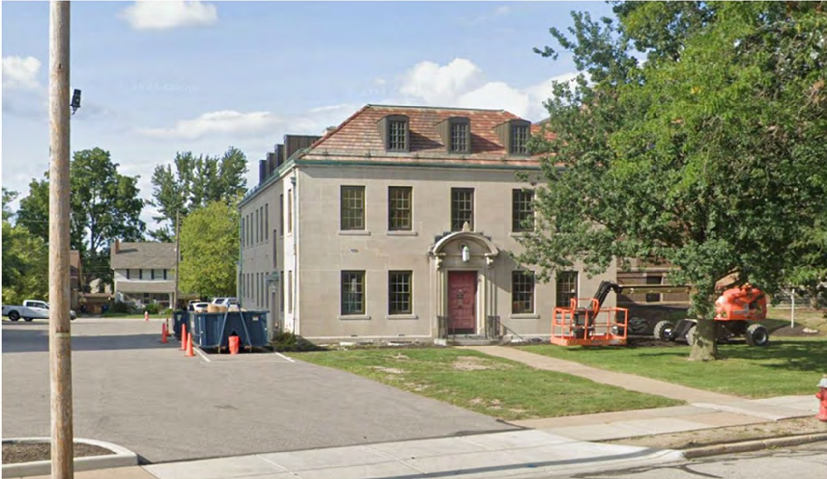
EXISTING BUILDING (PRE-RENOVATION) ALONG WITH LOCATION OF SIGN CONDITIONS
