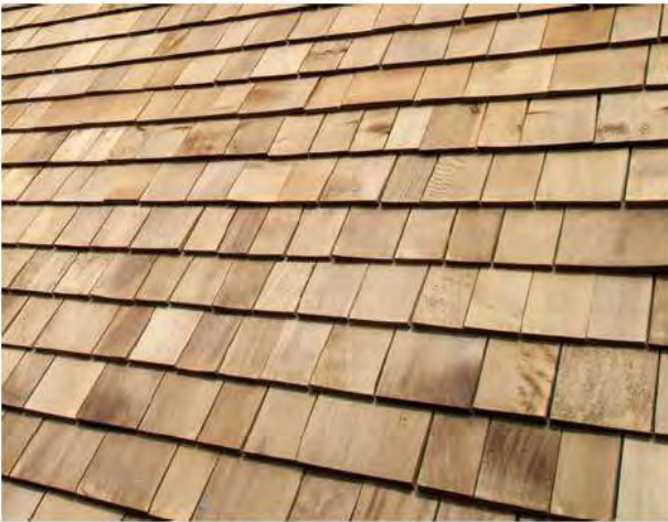
SHINGLES: CEDAR (TO NATURALLY WEATHER TO GREY)
