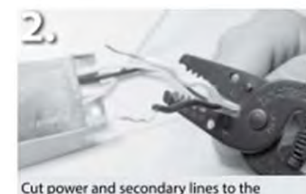
2. Cut power and secondary lines to the existing ballast and remove.
