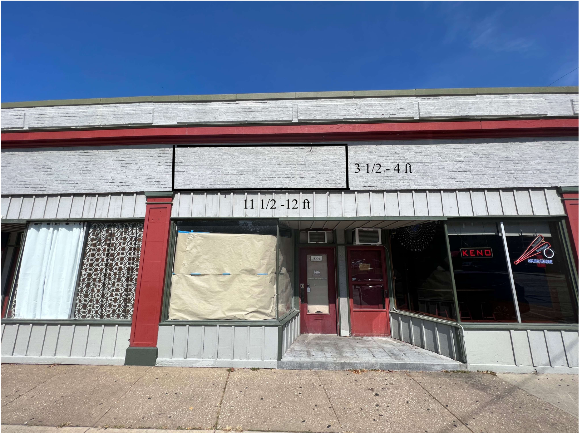
Docket No. 10-79-23 (13306 Detroit) Signage – Baadani Cloud City Vapes
