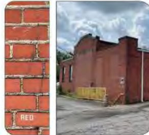
EXISTING BRICK, RED SMOOTH – EXTERIOR WALL BRICK
