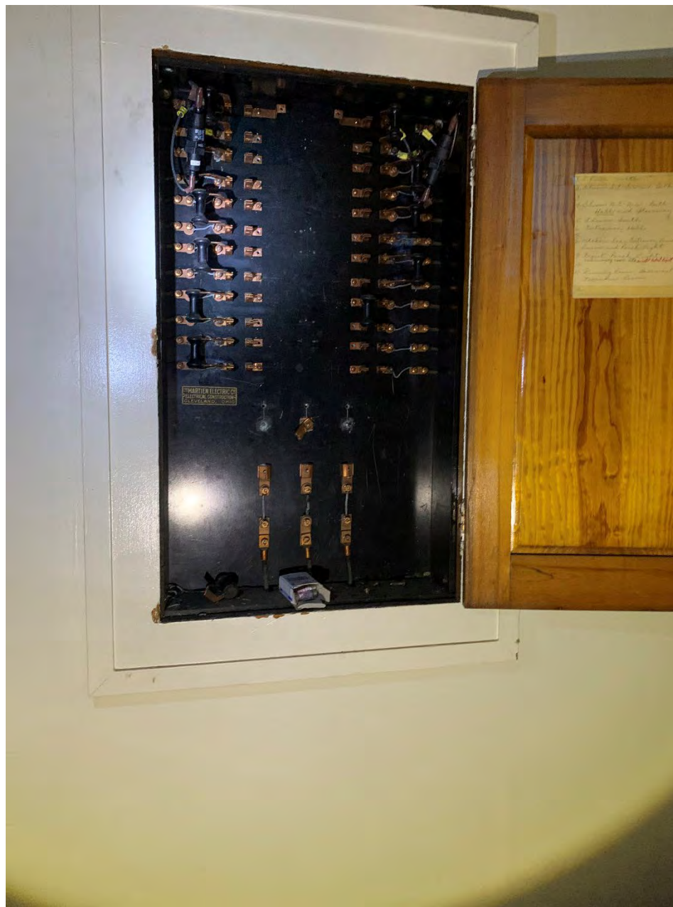
Docket No. 11-93-23 (12534 Lake) Demolition – Brummett Shady Cove Townhomes
