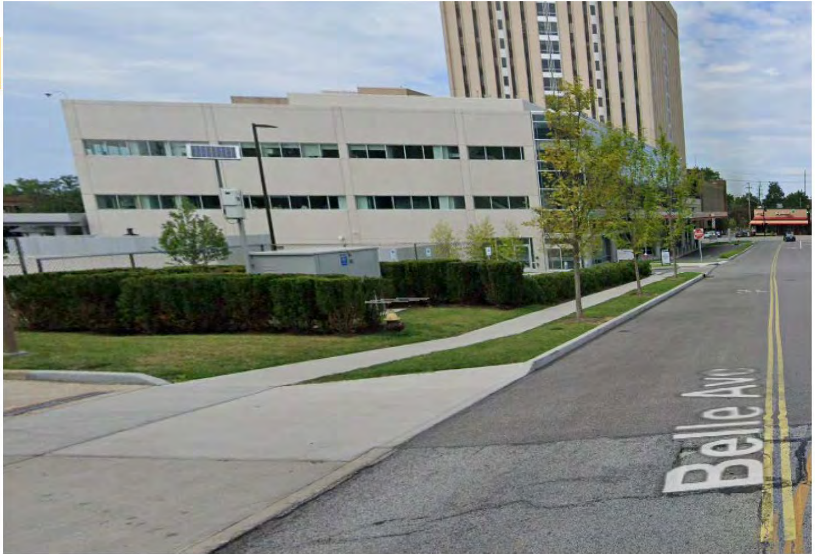
Family Health Center south elevation, facing the Lakewood Community Health Center
