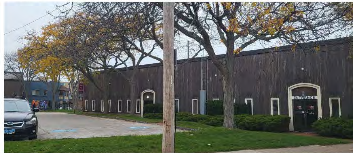
REAR OF EXISTING BUILDING
