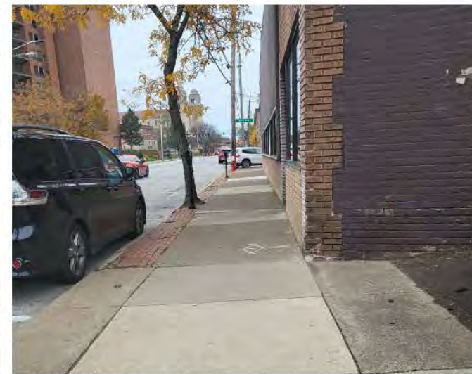
SIDEWALK ALONG DETROIT AVENUE
