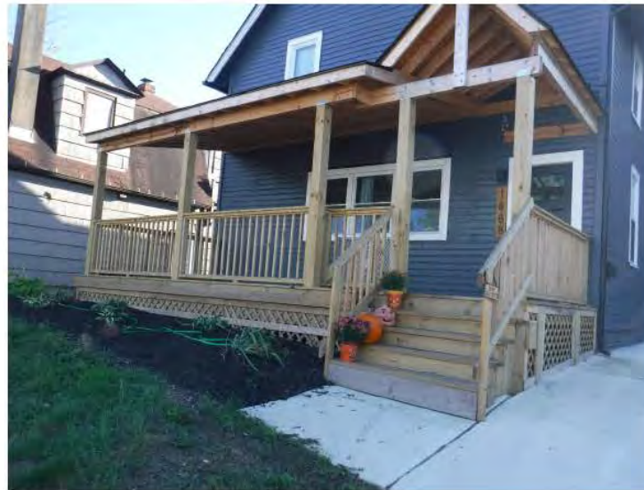
AS-BUILT FRONT PORCH VIEWING SOUTH
