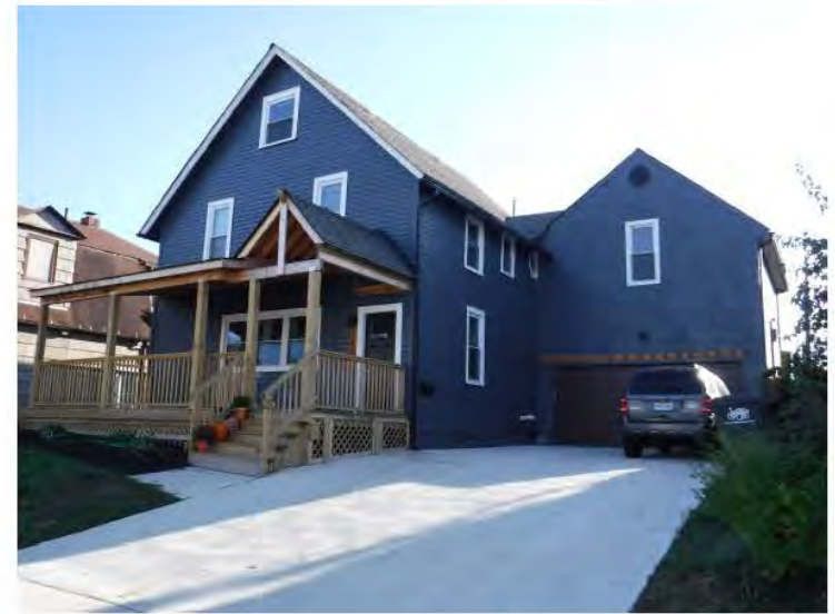
AS-BUILT VIEWING SOUTH
