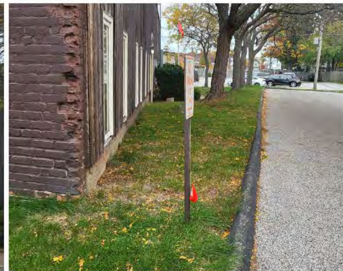
SLOPE BEHIND EXISTING BUILDING
