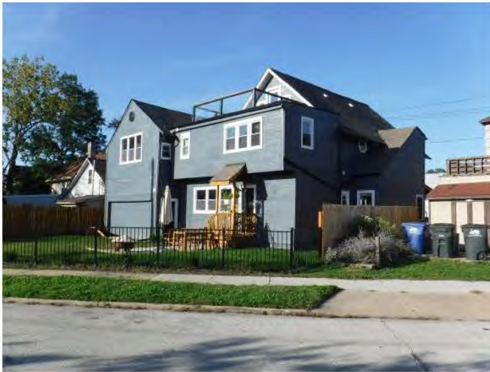
AS-BUILT VIEWING NORTH
