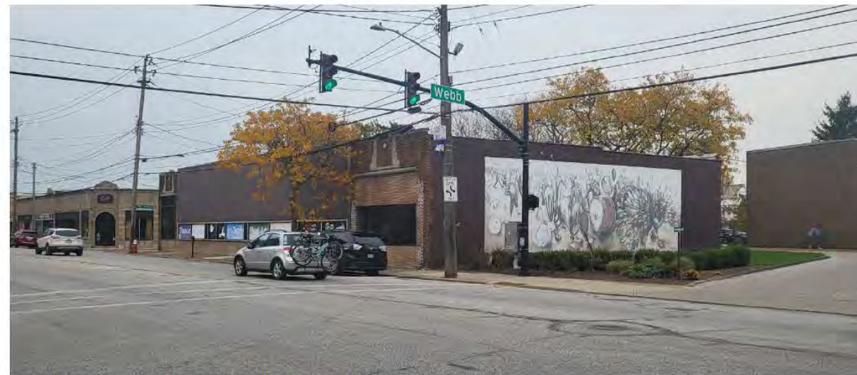
EXISTING BUILDING TO BE DEMOLISHED - VIEW FROM DETROIT AVENUE
