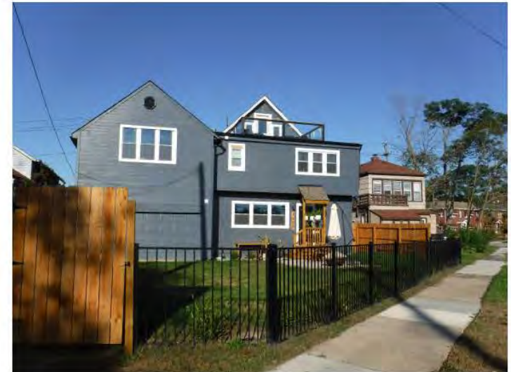
AS-BUILT VIEWING NORTHEAST
