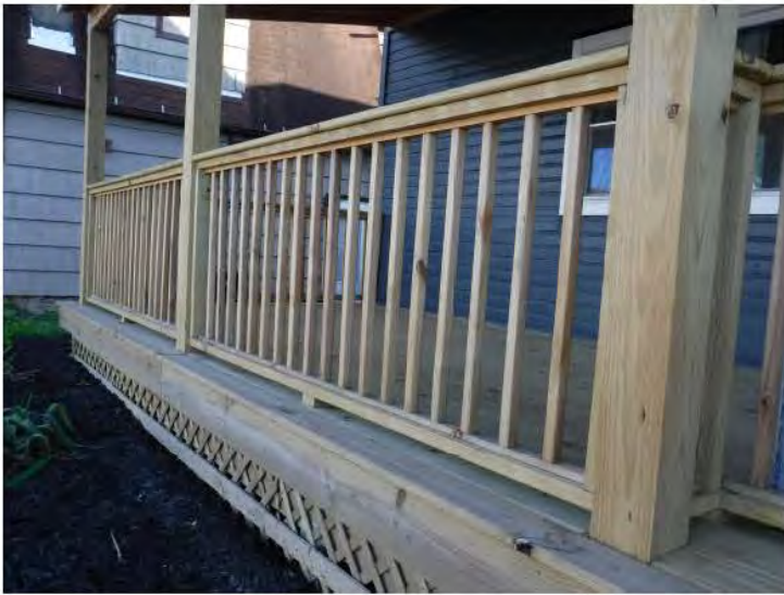
AS-BUILT FRONT PORCH RAILING
