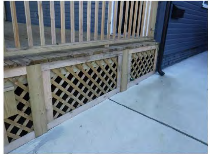
AS-BUILT FRONT PORCH LATTICE
