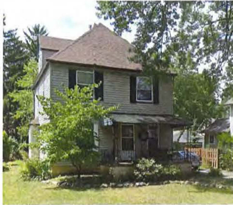
EXISTING FRONT PHOTO 1
