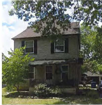
EXISTING FRONT PHOTO 2
