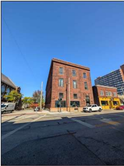
Front Photo Existing
