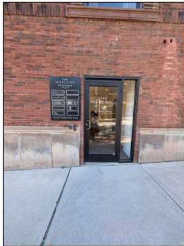
Marlowe Building Entry Door
