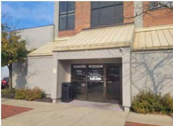
13 Remove existing 13000 & 13300 lettering. patch/ repair wood as required.
