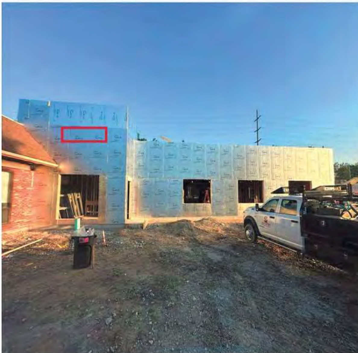
Exterior Foam Insulation Installed
