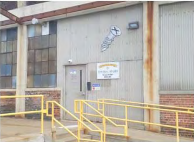
7 Remove existing Central Stair Signage and screw graphic.
