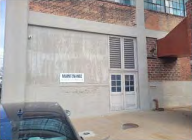
3 Remove existing Maintenance Parking Sign.
