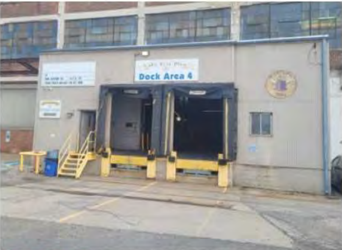
8 9 10 11 Remove existing Central Stair, Tenant, Dock Area 4, and Hawthorne Wire signage.
