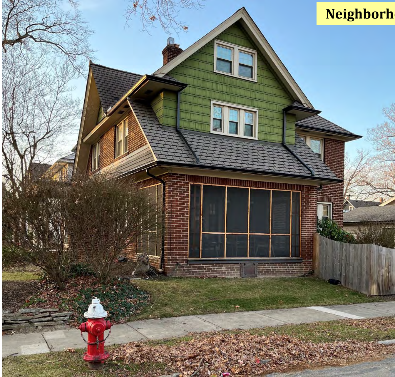
Docket No. 12-85-22 (1060 Abbieshire) Front Porch Screen Install
