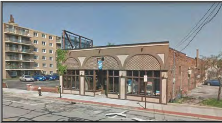
EXISTING CONDITIONS 1 FRONT (SOUTH) ELEVATION AT DETROIT SCALE: N.T.S.
