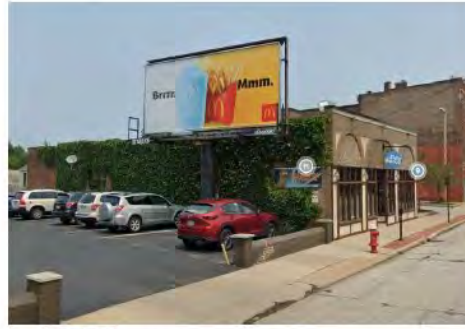
EXISTING CONDITIONS 2 FRONT (SOUTHWEST) CORNER AT DETROIT SCALE: N.T.S.
