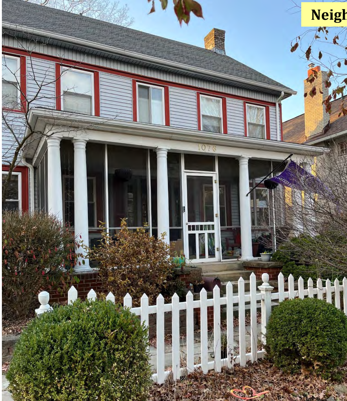
Docket No. 12-85-22 (1060 Abbieshire) Front Porch Screen Install
