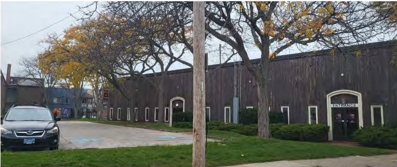
REAR OF EXISTING BUILDING
