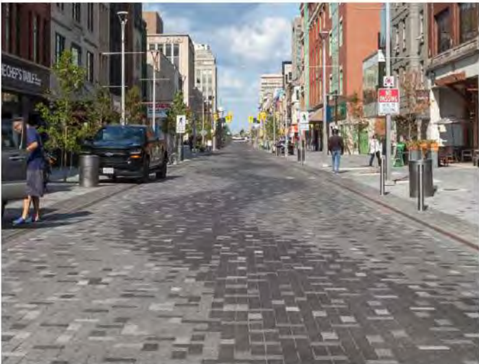
CURBSIDE DROP OFF WITH SERIES PAVERS FROM UNILOCK
