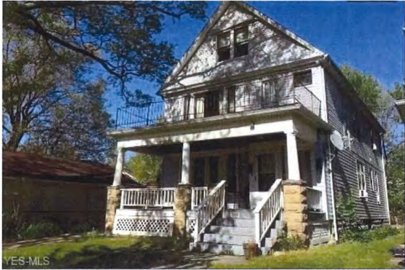
Prior Conditions - Second Floor Railing
