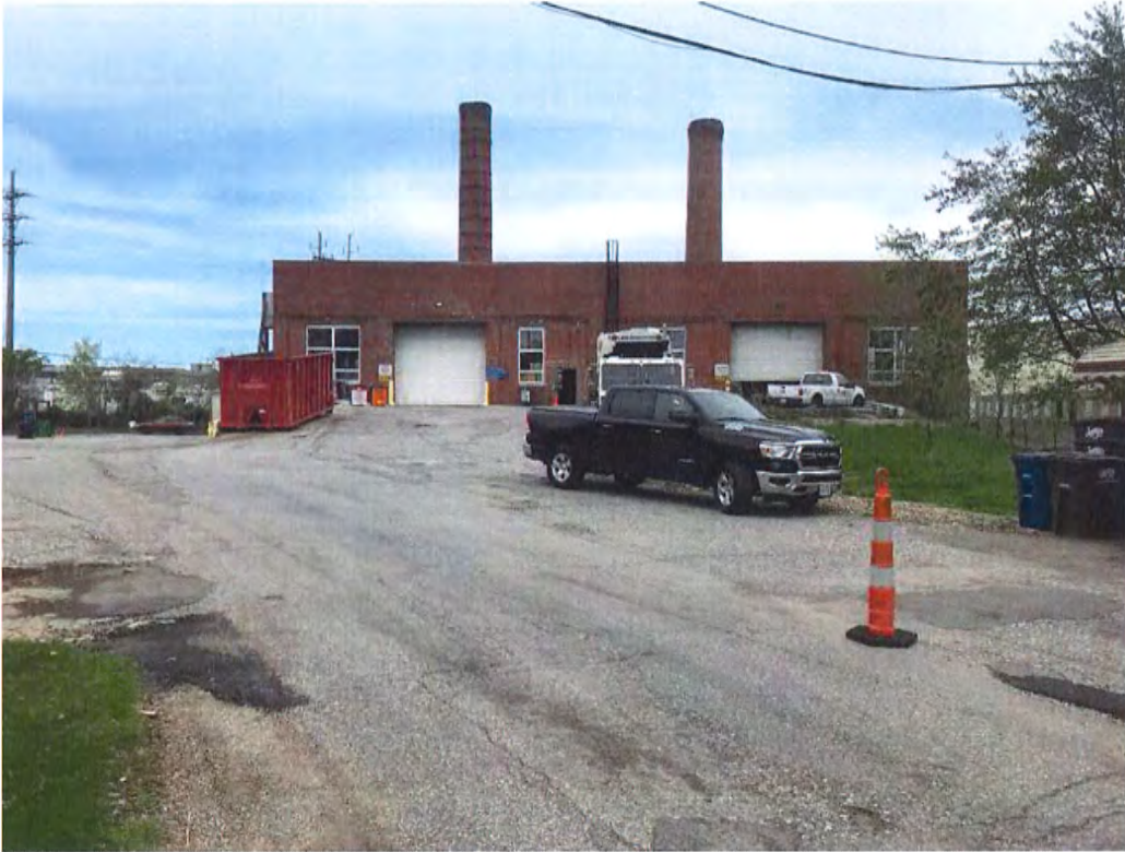
Picture 5: Existing Recycling Center (old incinerator bldg.) to be removed. Looking north
