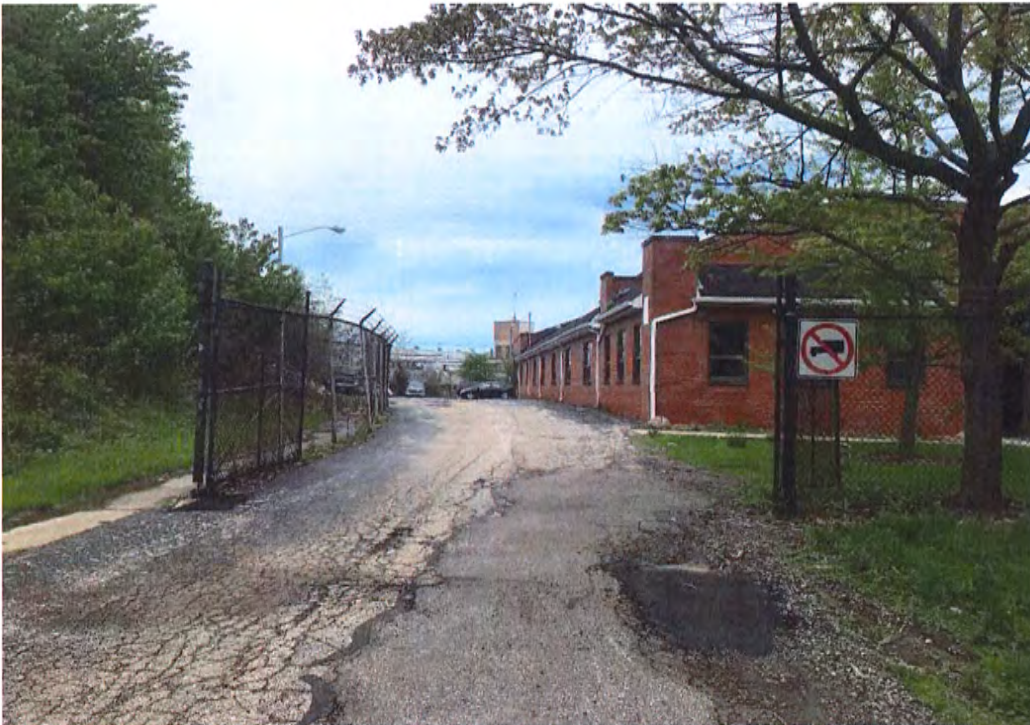
Picture 6: Existing Refuse Garage west side looking north from Berea Road
