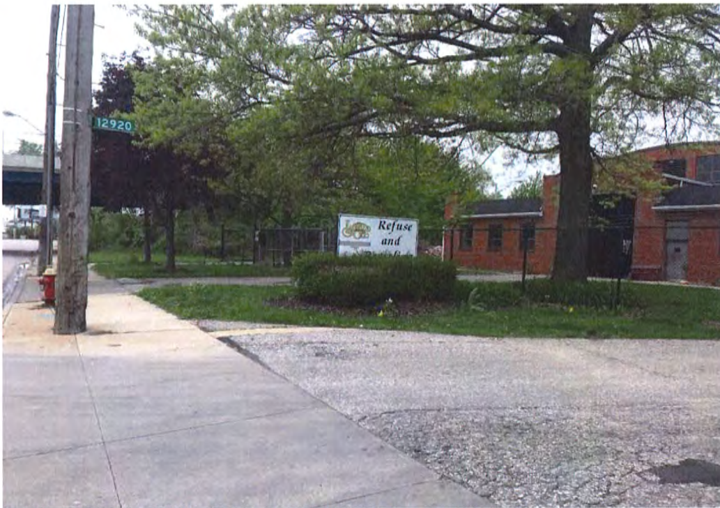
Picture 2: Existing Refuse Garage and Monument Sign along Berea Road looking west
