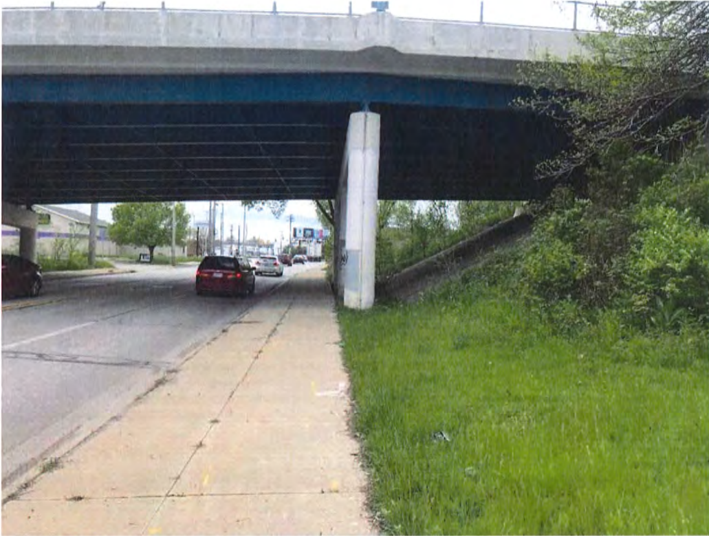
Picture 7: Lakewood Hts. Blvd. overpass west of property
