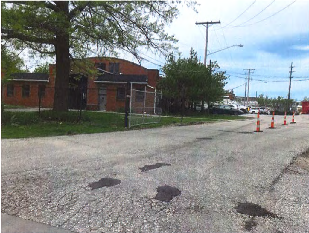
Picture 1: Existing Refuse Garage looking north from Berea Road entrance
