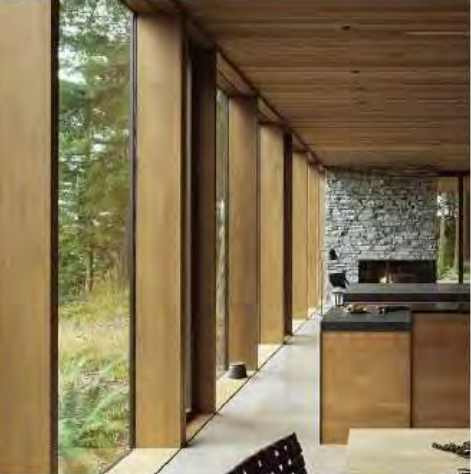
▲ Triple glazed curtain wall system
