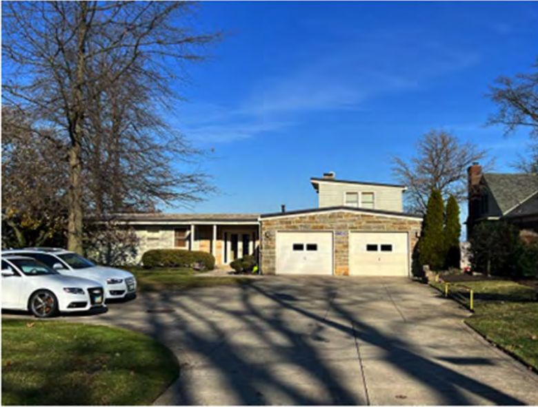
Existing structure, as seen from Edgewater Drive
