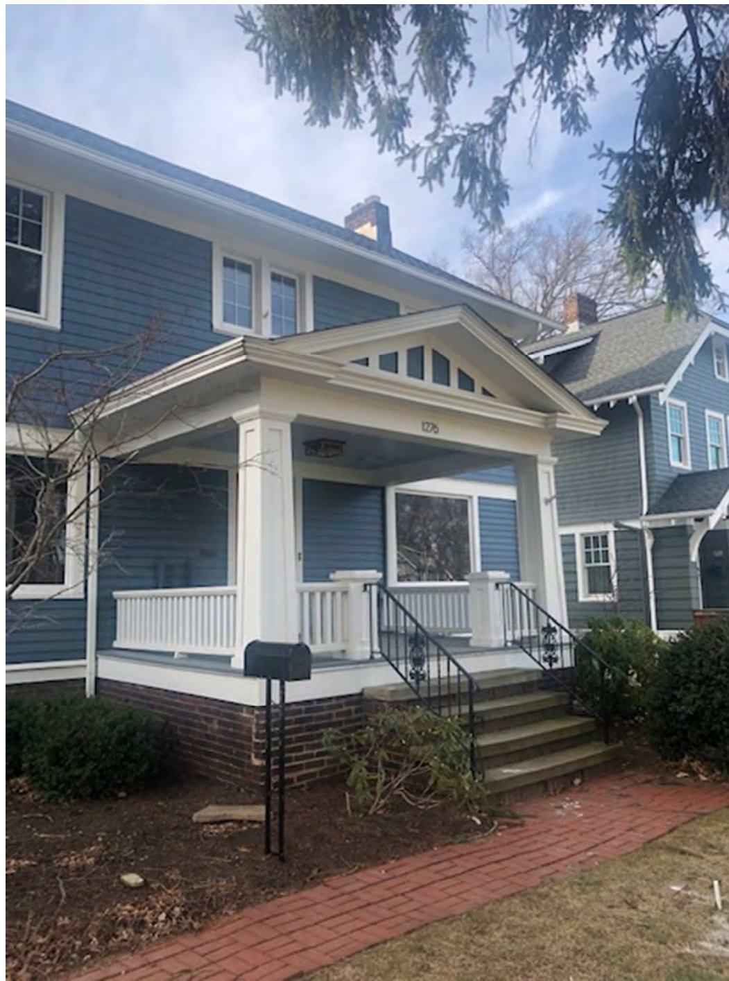
Docket No. 4-22-24 (1276 Manor Park) Residential Renovation - Brandt
