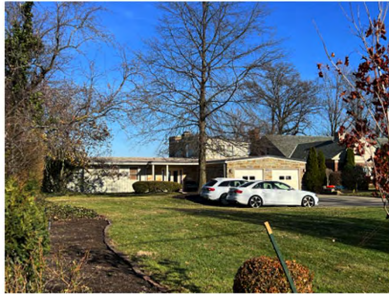
Existing structure to be demolished
