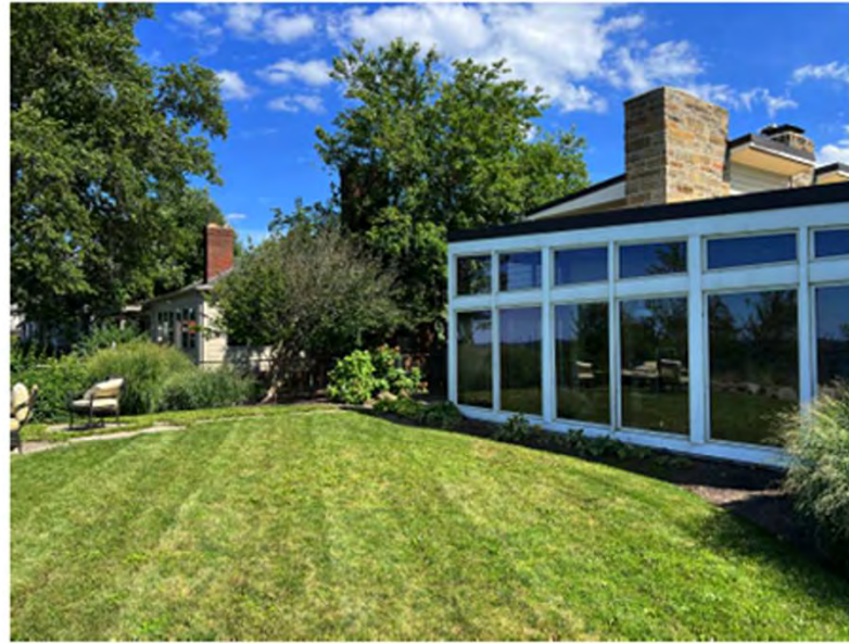
Existing structure showing green buffer and neighbor to the East
