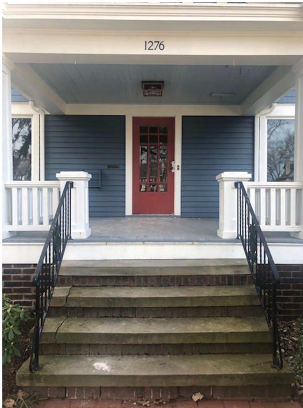
Docket No. 4-22-24 (1276 Manor Park) Residential Renovation - Brandt
