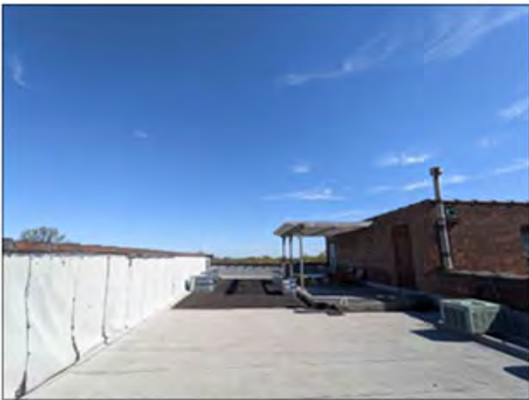
Existing Accessible Roof
