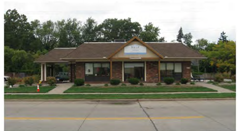
SOUTH (FRONT) WALL LOOKING NORTH FROM SLOAN AVE
