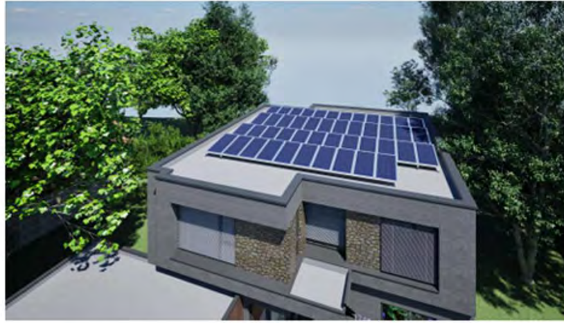
Concealed solar panels
