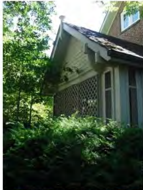
EXISTING PHOTO VIEWING SOUTHWEST
