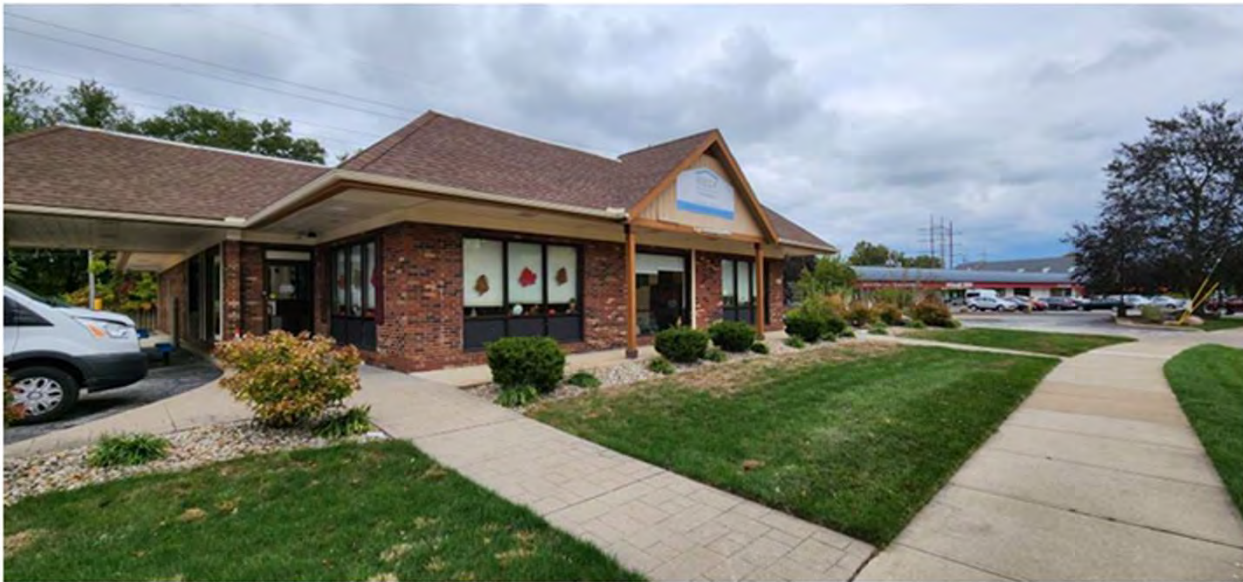
EXISTING BUILDING FROM SOUTHWEST
