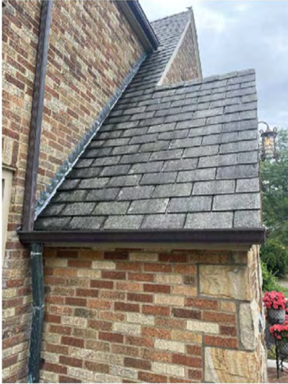
Existing Brick & Roofing
