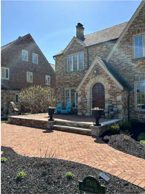
Existing Patio - From West
